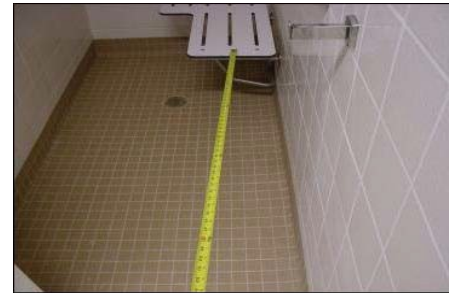
Men's Locker Room
