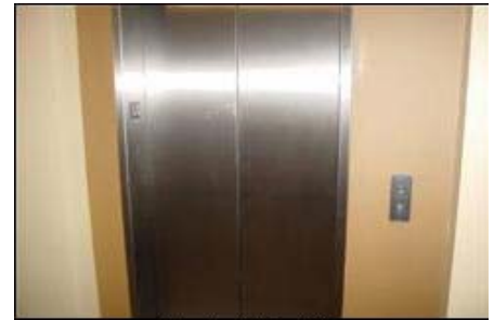
Elevator in Main Lobby
