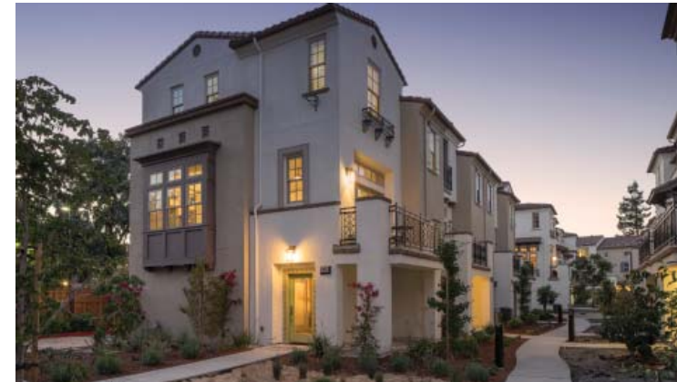
Example of porch used as a ground floor projection
