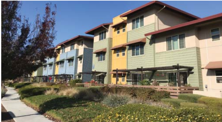
Example of fencing at individual yards to enclose the space and provide privacy
