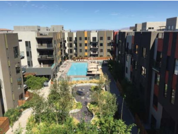
Example of a resident amenity located on top of a podium
