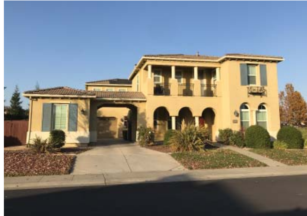
Example of the garage located in the rear of the lot
