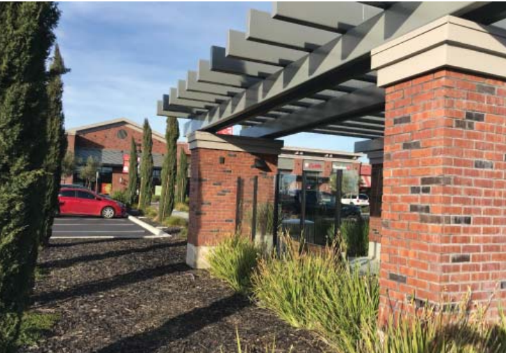
Example of a pedestrian path providing safe and easy access to buildings
