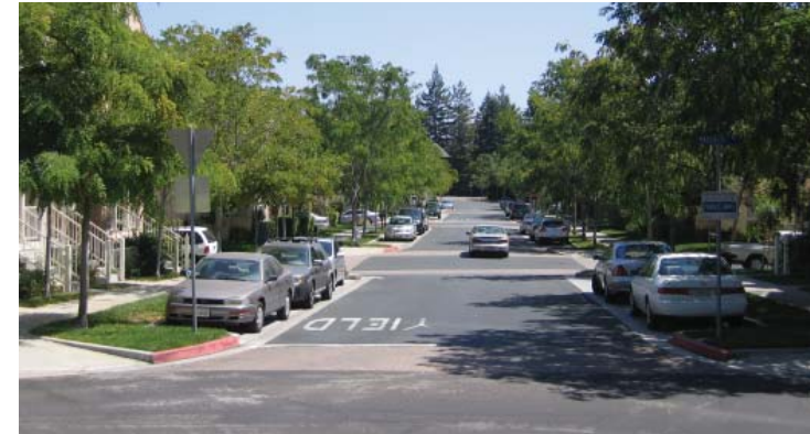
Example of a bulb-out on a residential street to slow traffic
