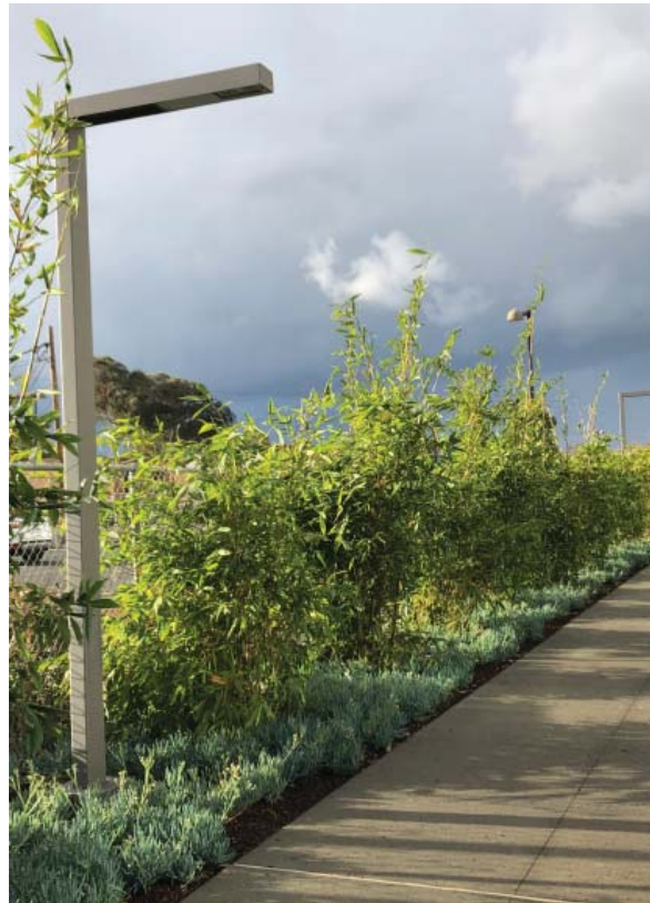
Pedestrian scaled downward directing light fixture
