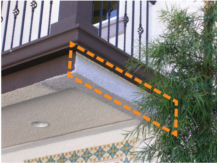
NOT RECOMMENDED: Example of how colors should shall not terminate on outside corners
