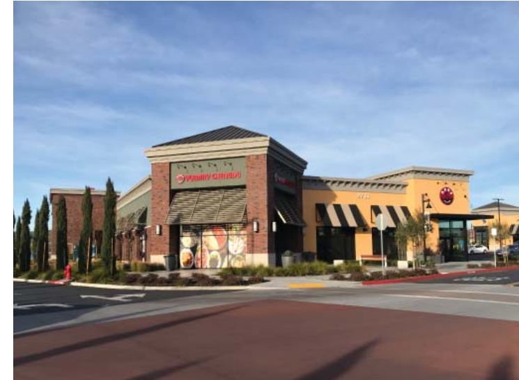
Tower elements should be used as gateways to create a sense of place
