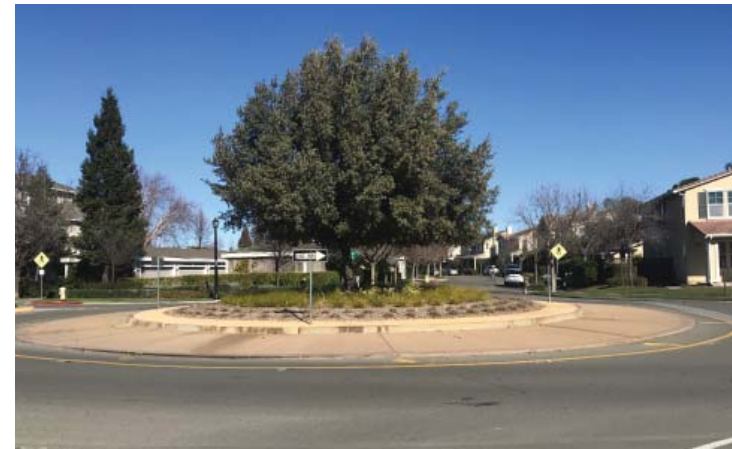
Example of a traffic circle as a traffic calming tool
