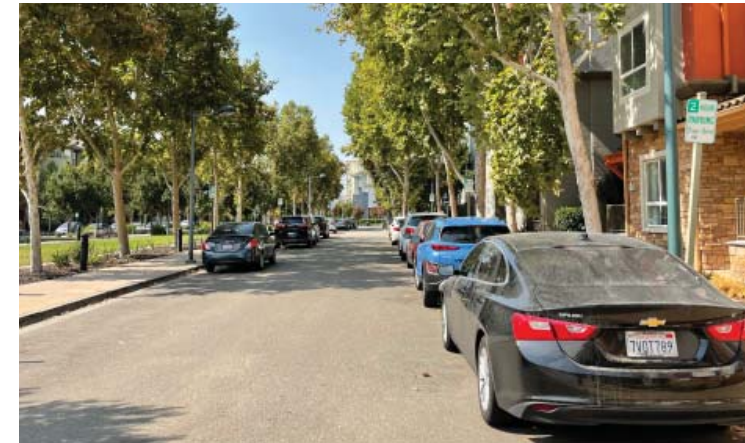
Example of a narrow one-way street used for traffic calming
