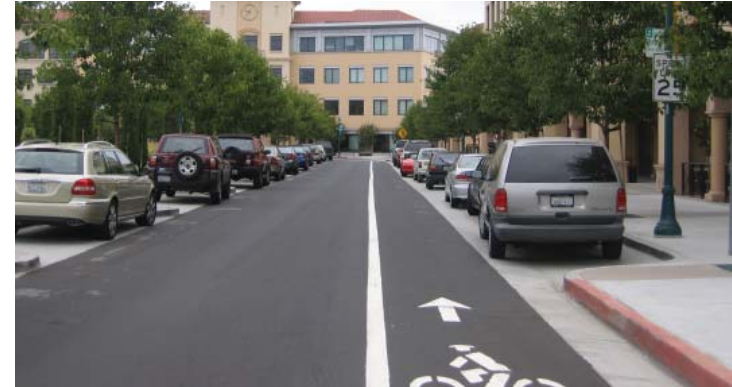
Example of an on-street bike lane
