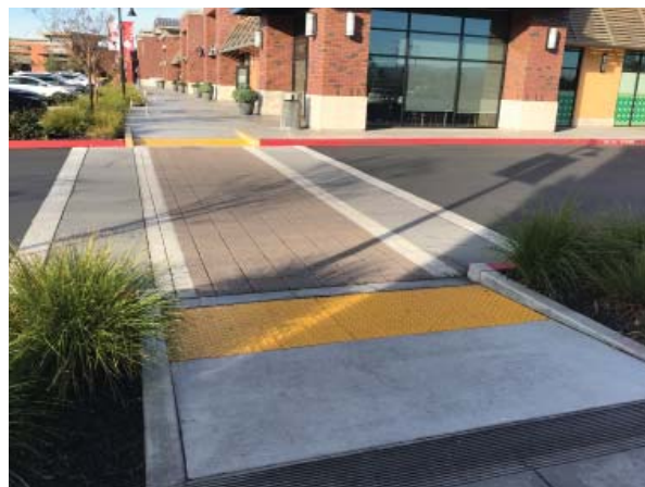
Incorporate a change in material or pattern to highlight pedestrian routes through drive aisles
