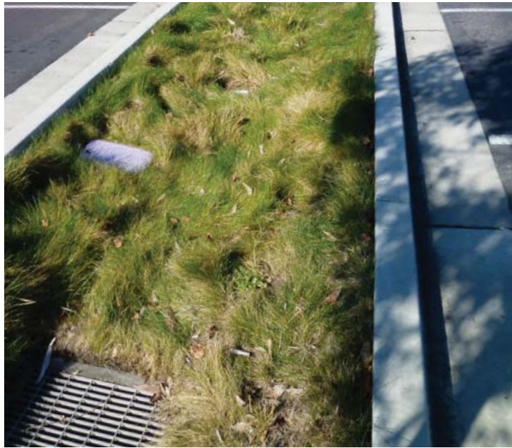
Techniques for stormwater treatment shall be utilized
