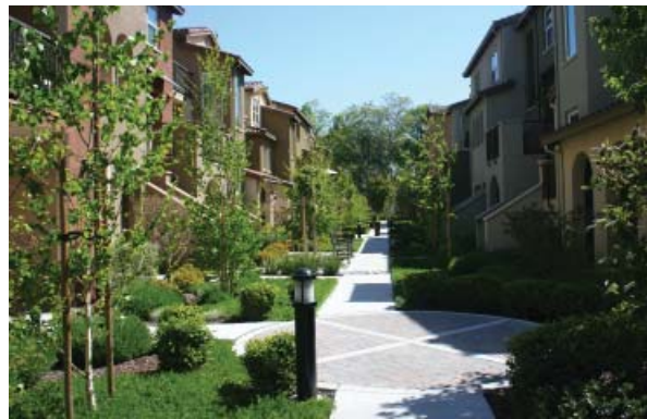
Example of a clear and visible pedestrian pathway
