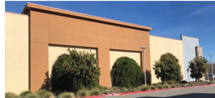
Blank façades should be avoided through change in planes, materials, colors, and landscape
