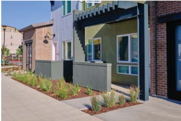
Example of low walls at unit entires to create privacy and security
