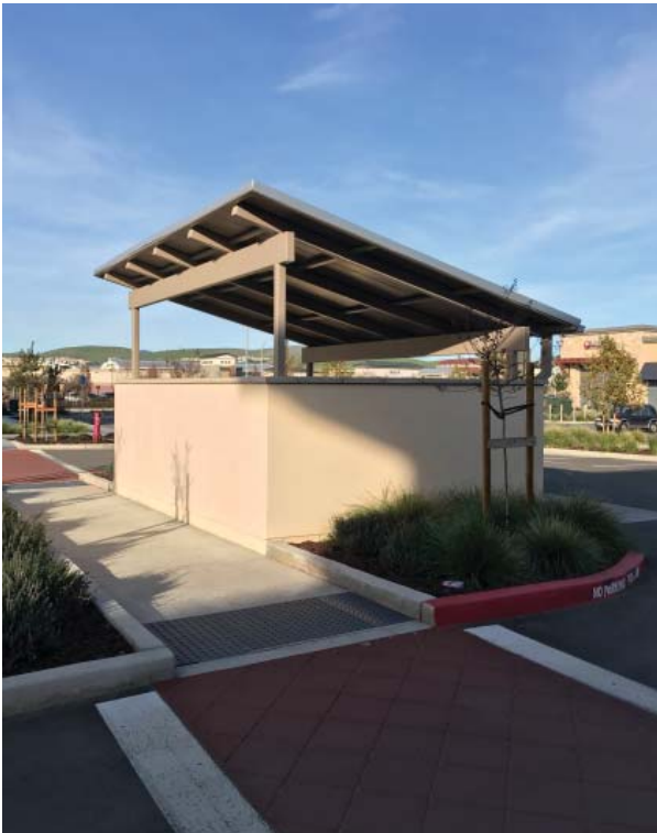
Trash enclosures shall have a clear path of travel for ease of access
