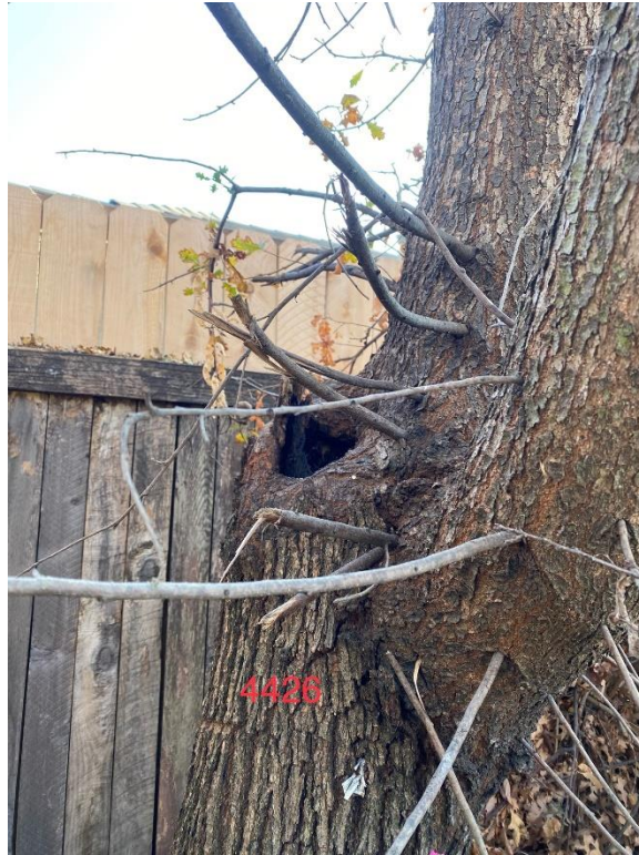
Tree #4426 showing proximity to fence, cavity on north side and weak branch attachment.
