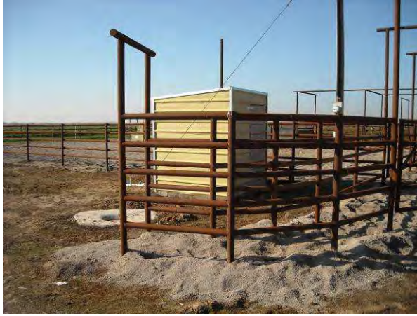
P12-SW: View of the covered structure surrounding the well in the northeastern corner of the property.
