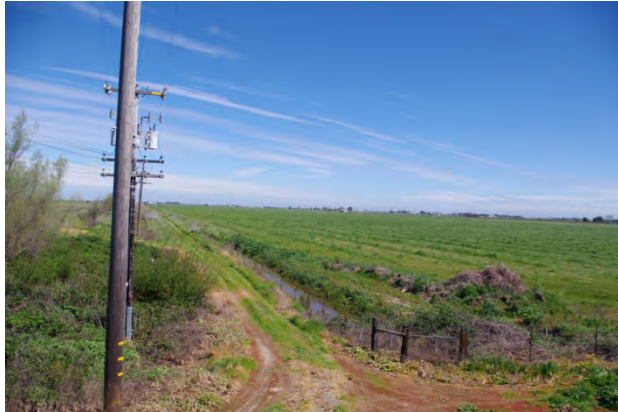
P10-N: View of the western border of the property, taken from the levee road.
