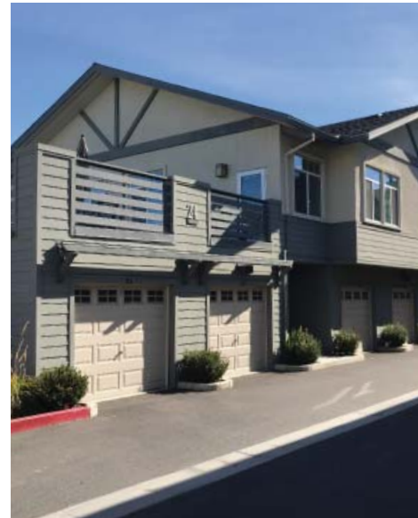
Example of the use of garage doors to provide contrast
