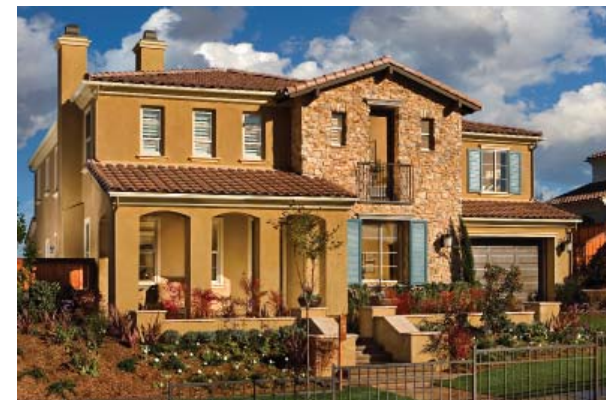
Example of chimney located on an internal wall away from street view
