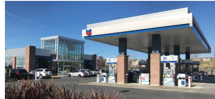
Service station canopies should compliment the building character
