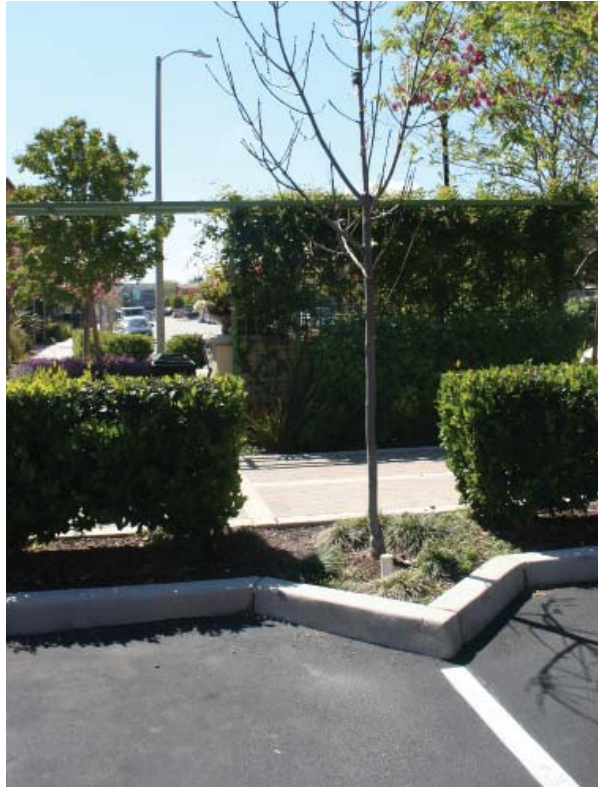
Trees shall be protected from vehicle damage by a minimum six-inch curb
