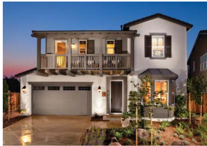
Example of balcony cantilevering over the garage
