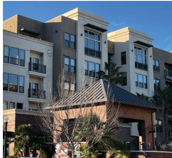
Example of a facade break
