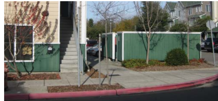
The color and material of trash enclosures shall match the style of the buildings
