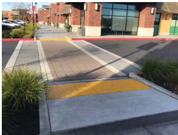
Incorporate a change in material or pattern to highlight pedestrian routes through drive aisles
