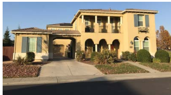
Example of the garage located in the rear of the lot
