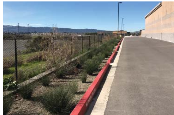
Open fencing shall be used when the project is adjacent to open space
