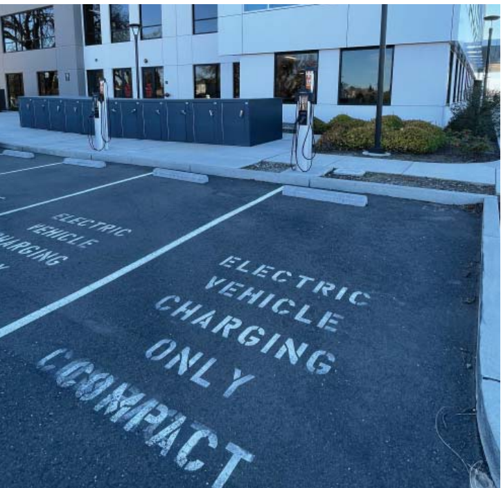
Electric Vehicle (EV) charging stations and bike lockers within parking lots
