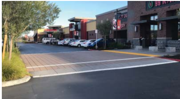
Raised crossings (tabletops) or change in material to highlight pedestrian crossings are encouraged in front of major entries
