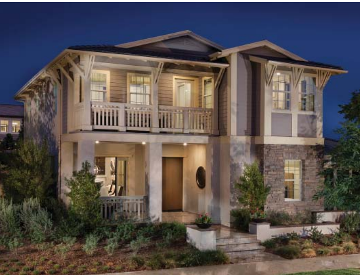
Example of incorporating a minimum 5x8 foot porch on the front entry
