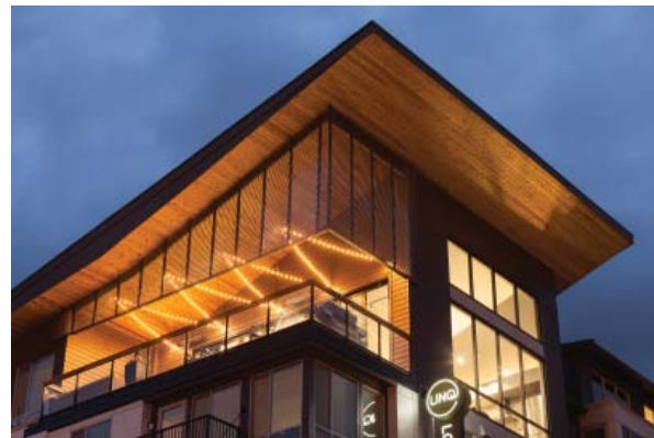
Example of building lighting to highlight specific building components
