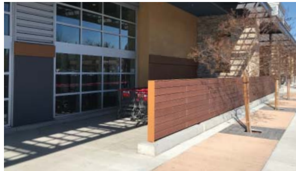
Screen shopping cart return areas when adjacent to the building
