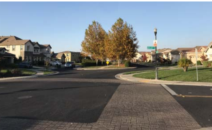
Incorporate visual cues for pedestrian crossings such as a change in pavement
