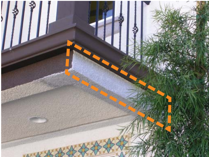
NOT RECOMMENDED: Example of how colors should not terminate on outside corners
