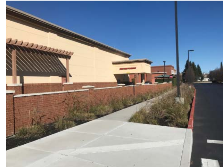
Walls can lower the impact/appearance of a drive-through
