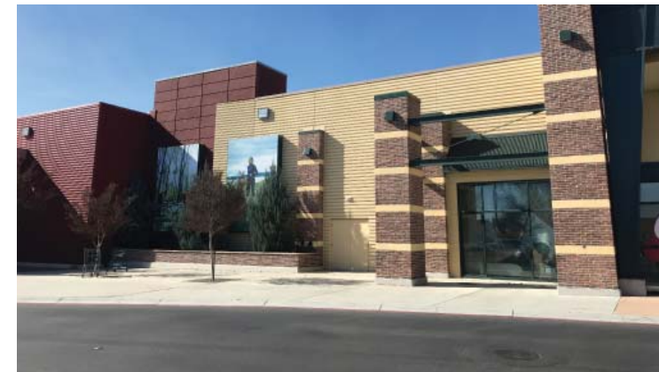
Color and material should be used to break up the massing of the building
