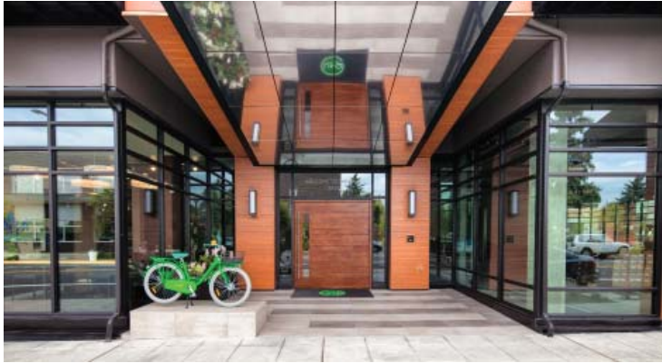
Example of an easily identifiable main building entry
