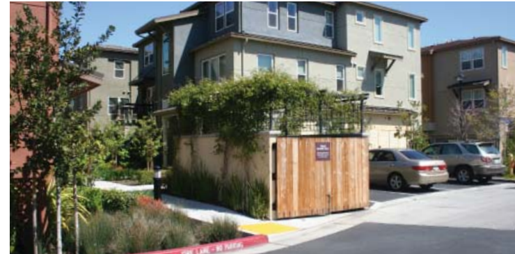
Example of a well screened trash enclosures
