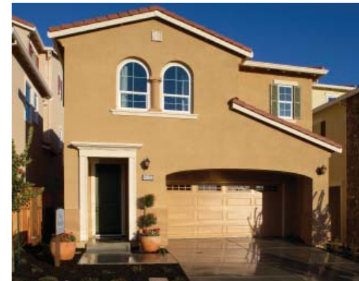
Example of a recessed garage door created the by extending the upper story
