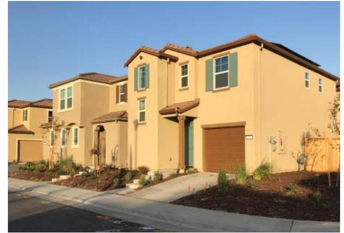
Example of a single car garage door use
