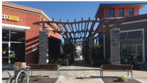
A visual link between buildings shall be provided, in this case a trellis
