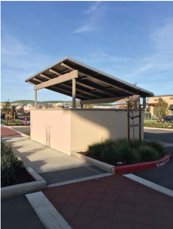
Trash enclosures shall have a clear path of travel for ease of access
