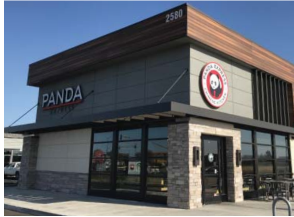
Entries shall be clearly defined and within the same scale of the project
