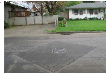
Figure 1. A UIC located in a public right of way. Source: Oregon DEQ UIC program.
