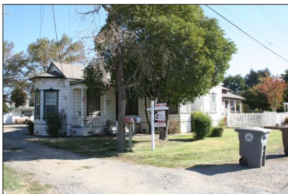
Figure A: Front building at 9081 Grove Street (GPA, September 2018)
