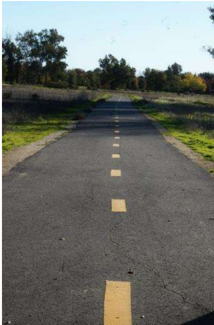
Figure 28. No speed stencils, signs, or other markings are present that might help pedestrians and bicyclists understand how best to share the trail.
