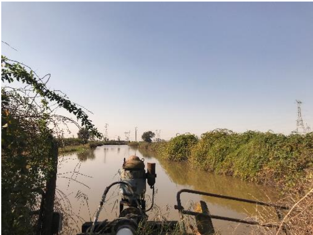
Deep retention pond, Kendrick Parcel, facing west. 28 September 2020.
