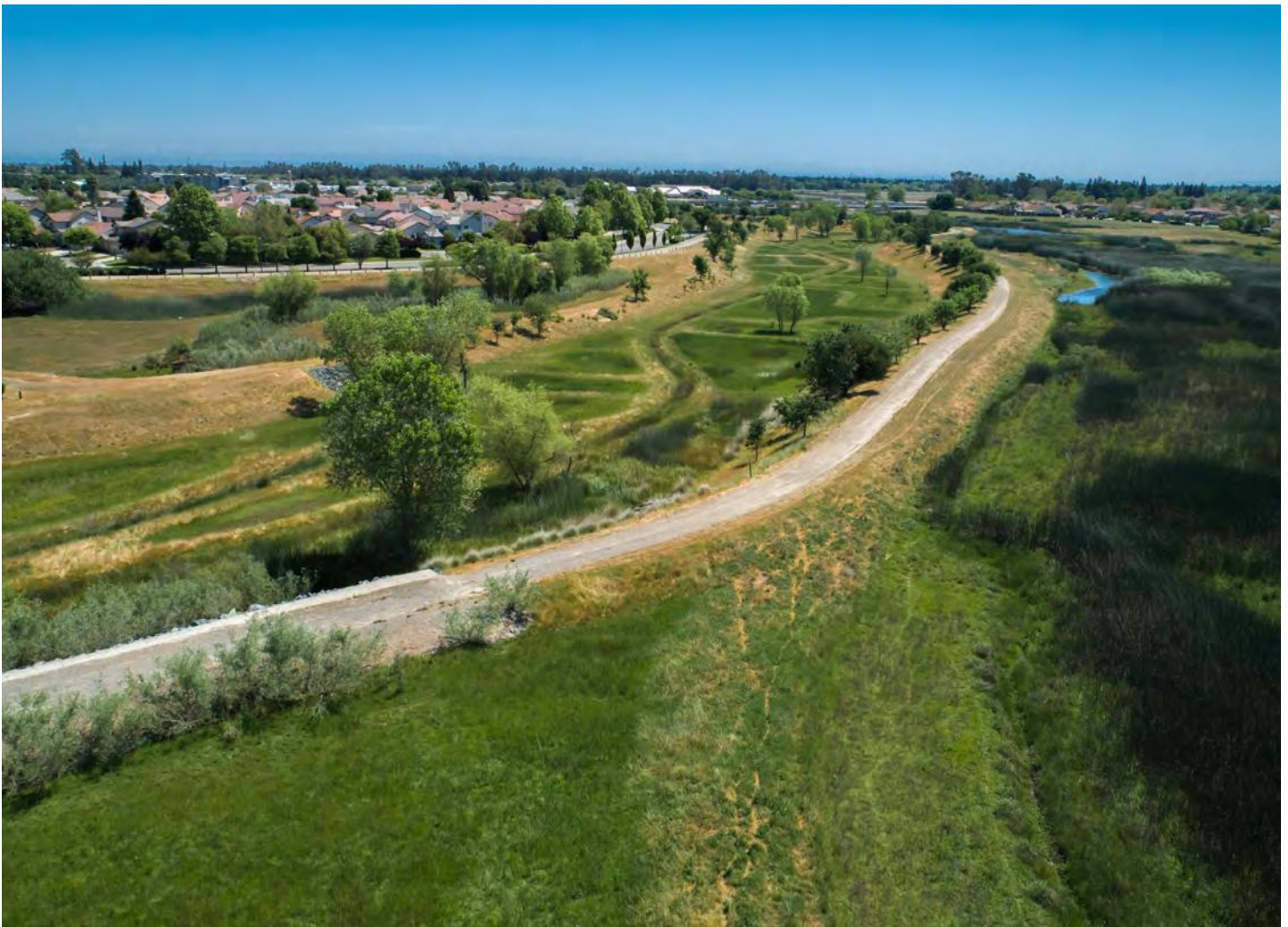
Elk Grove Creek in the north east portion of the City
