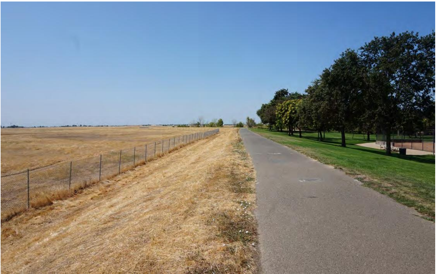
Laguna West Levee System near Don Nottoli Park
