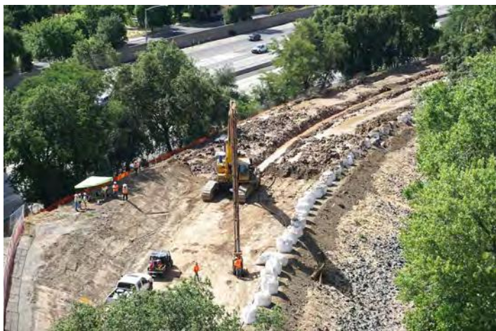
U.S. Army Corps of Engineers construct cutoff wall to reduce seepage and stability issues along the Sacramento River East Levee
