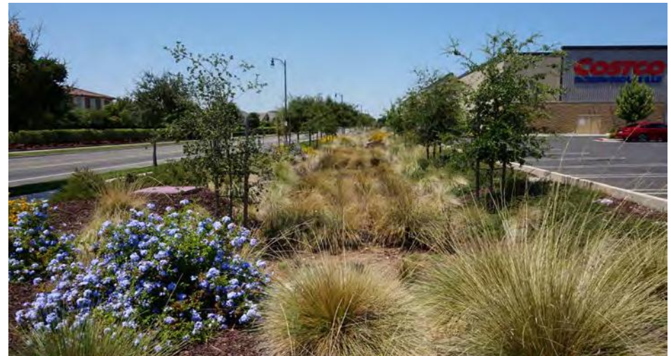
Bioswales and other green infrastructure can help reduce localized flooding impacts, improve water quality, and mitigate the UHI effect.
