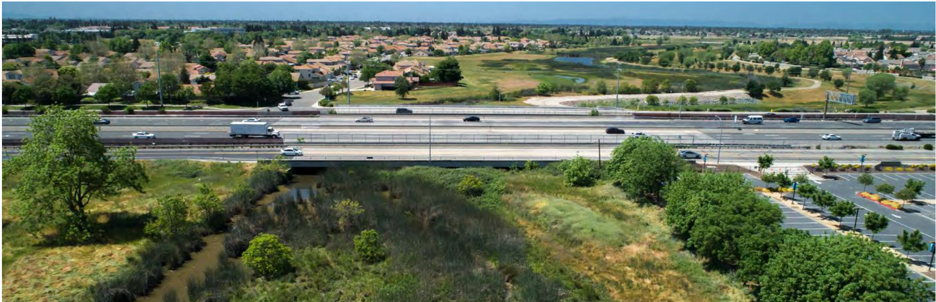
State Route 99 bridge over Elk Grove Creek.
