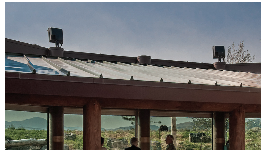
Habitat illumination via shade structure mounted gobo projectors with visors. Where surrounding structures are not tall enough and there are no appropriate trees for moonlighting, discrete poles with will be utilized for mounting.
