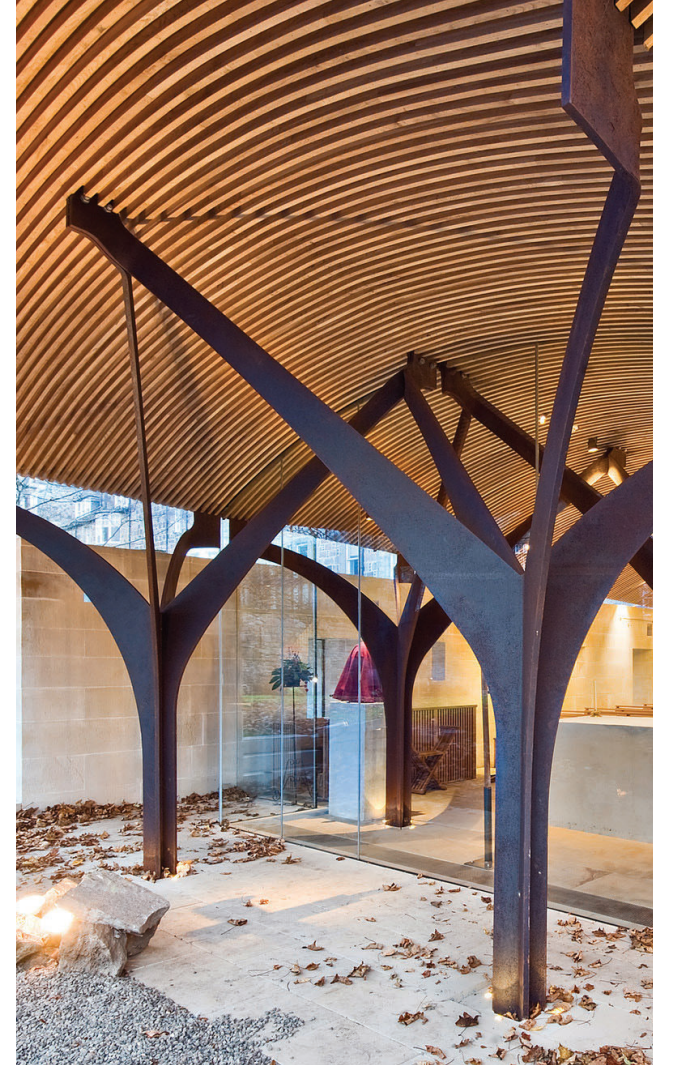
Up lighting at the base of the tree columns to highlight them as a feature and glow the ceiling canopy.
