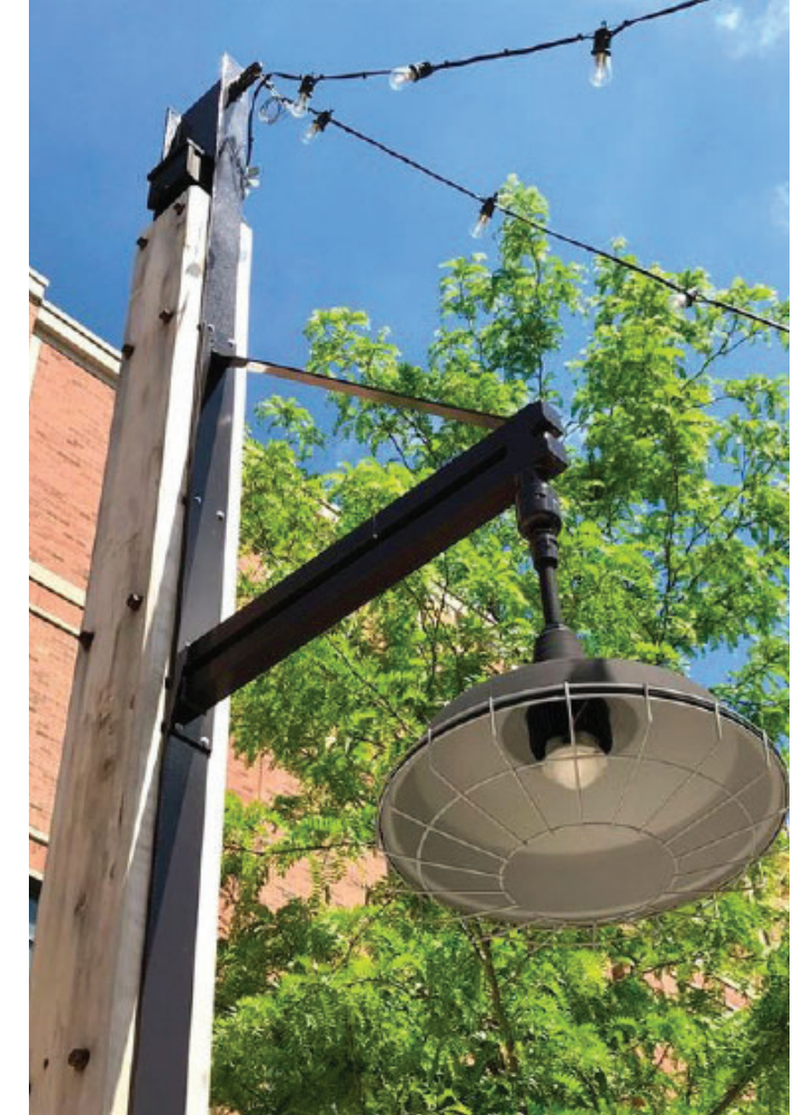
Pole mounted RLM shades for general illumination in open areas.
