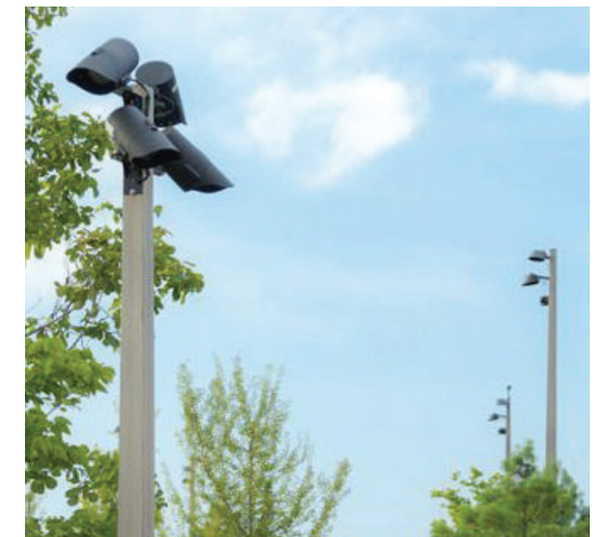
Habitat illumination via shade structure mounted gobo projectors with visors. Where surrounding structures are not tall enough and there are no appropriate trees for moonlighting, discrete poles with will be utilized for mounting.
