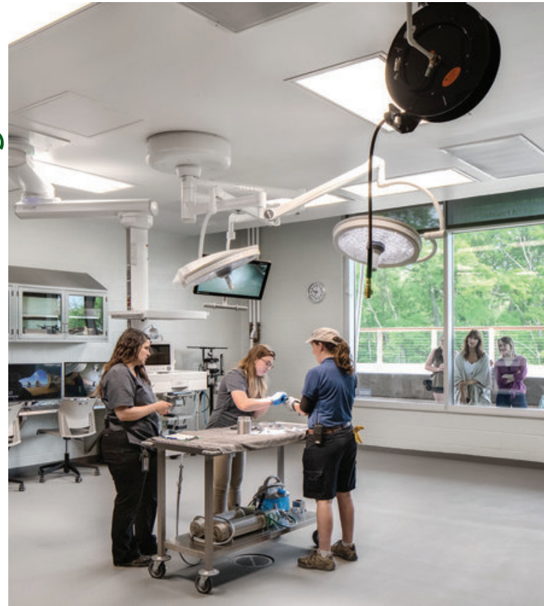
Gasketed low-glare recessed lighting for Animal Care Lab and Treatment rooms.
