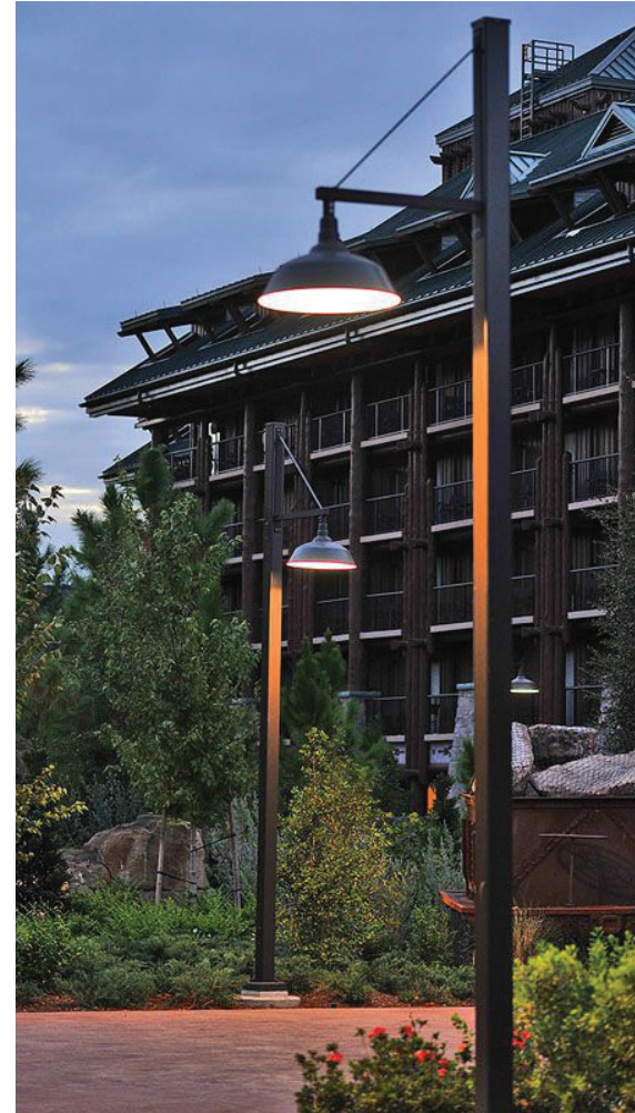
Pole mounted RLM shades for general illumination in open areas.
