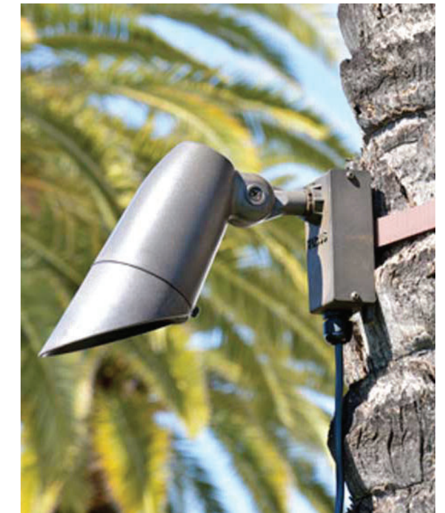
Adjustable luminaires mounted in trees for a downward moonlighting effect at large feature trees along main pathway.
