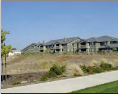
Photo IV-1: This multi-family project is scaled down at the edges of the property where it is adjacent to single-family development along the far property line.
