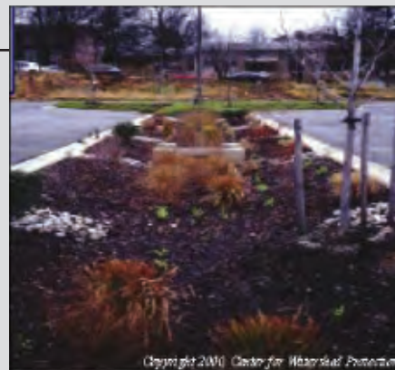
Photo V-22: Parking lot planter with intermittent curb cuts to allow parking lot runoff to drain into landscape area.
