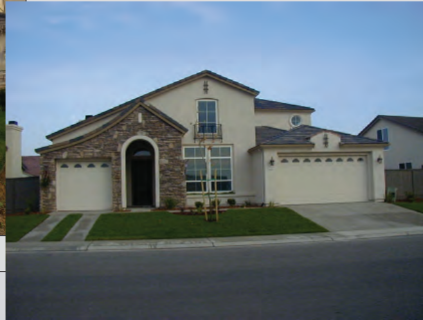
Photo III-71: Third and fourth car garage is perpendicular to street with window articulation , announcement of entry, and driveway width is limited to 16 feet
