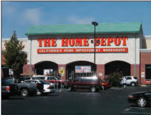
Photo V-62: This variation in roof design, as well as building offset, creates a focal point at the primary entrance to this larger building.
