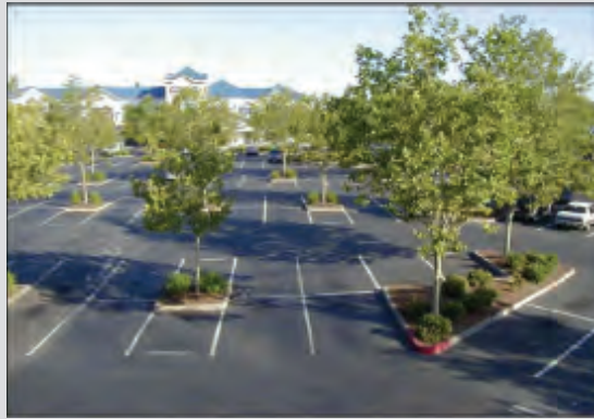
Photo V-20: Tree planting throughout this parking lot has been designed to meet minimum shade requirements.
