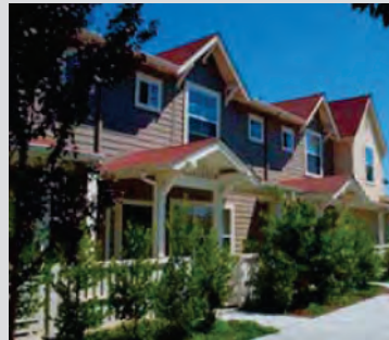
Photo IV-31: The entries to individual units are identified by the use of large dormered roof overhangs, landscaping, and pedestrian walkways.
