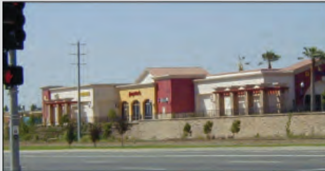
Photo V-33: The rear building facades facing the street include substantial offsets in the wall planes, variations in roof plans, and a combination of windows, landscape structures, and contrasting colors.
