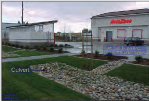
Photo V-19: Perimeter planter area designed with a drainage swale to capture urban runoff from the parking area.
