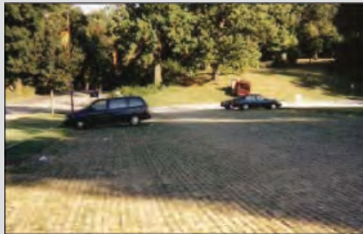
Photo V-16: This photo shows an alternative parking lot paving surface that is porous.
