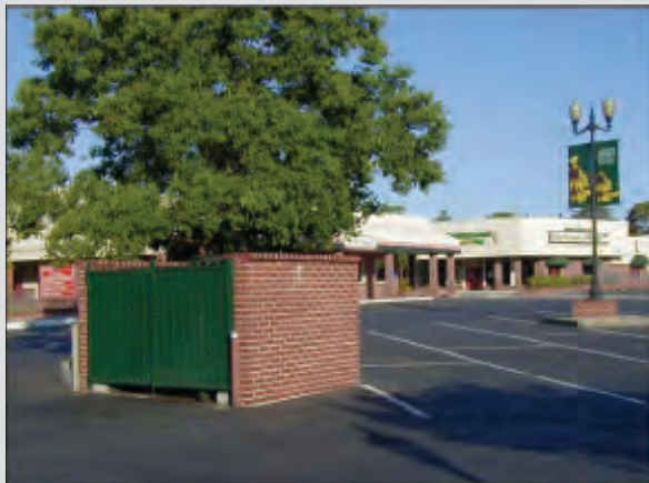
Photo V-29: This photo shows trash-enclosure materials and colors that match the adjoining development.
