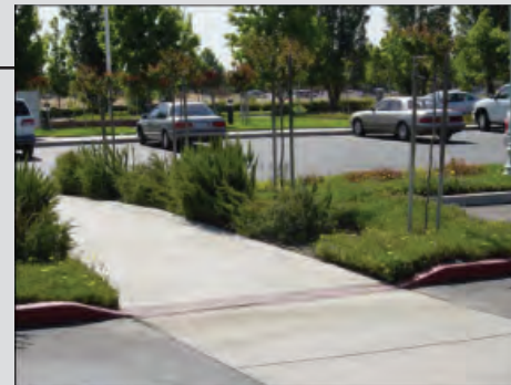
Photo V-26: This pedestrian walkway through a landscape planter is well designed as a visible and convenient crossing intended to avoid damage to the landscaping.
