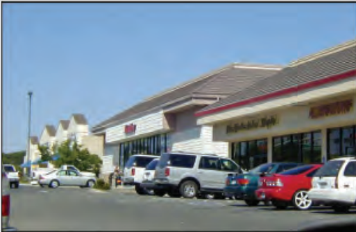
Photo V-52: This photo shows the distant building with roof features that are applied rather than incorporated as shown in the foreground buildings
