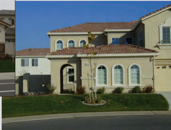
Photo III-73: Third car garage is perpendicular to street with window articulation and announcement of entry
