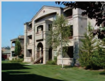
Photo IV-30: Entrances to individual units are clearly delineated by the use of arched entryways.
