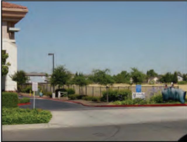
Photo V-8: Openview fencing behind a commercial center in Elk Grove.
