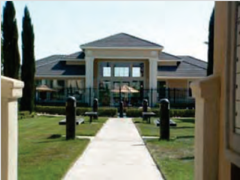
Photo IV-18: Bollard lighting is used to illuminate a pedestrian walkway within this multi-family project.
