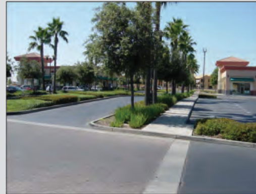
Photo V-10: Special pavement used to highlight pedestrian walkways and for traffic calming within a commercial center in Elk Grove.
