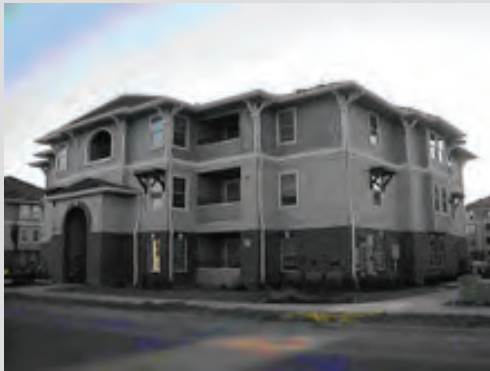
Photo IV-19: This multi-family project has a Craftsman style of architecture with characteristic elements on all elevations.
