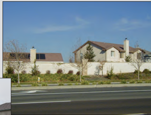
Photo III-23: Masonry soundwall with trim cap, softened by landscape screening
