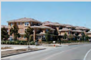
Photo IV-21: Mass and scale of a multi-family project can be reduced by the use of varied roof patterns and recessed facades.
