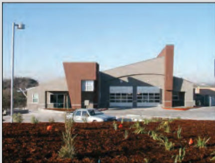
Photo V-64: This concrete fire station utilizes interesting building forms and colors to create visual interest.
