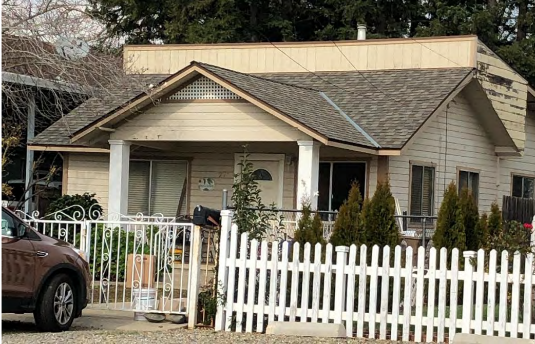
Photograph 1. View northwest of the south and east elevations.
