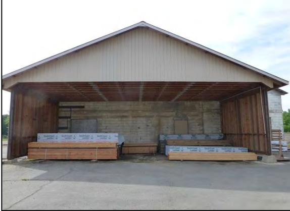
Photograph 15. North elevation of Bldg. 4 with an affixed 1984 addition. Camera facing south.
