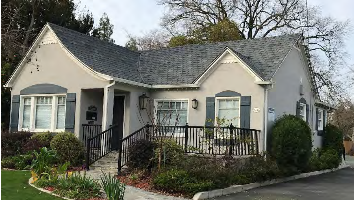
Photograph 1. View northwest of the south and east elevations.
