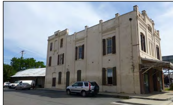
Photograph 5. Overview of warehouse (left) & IOOF Hall (right). Camera facing northeast.
