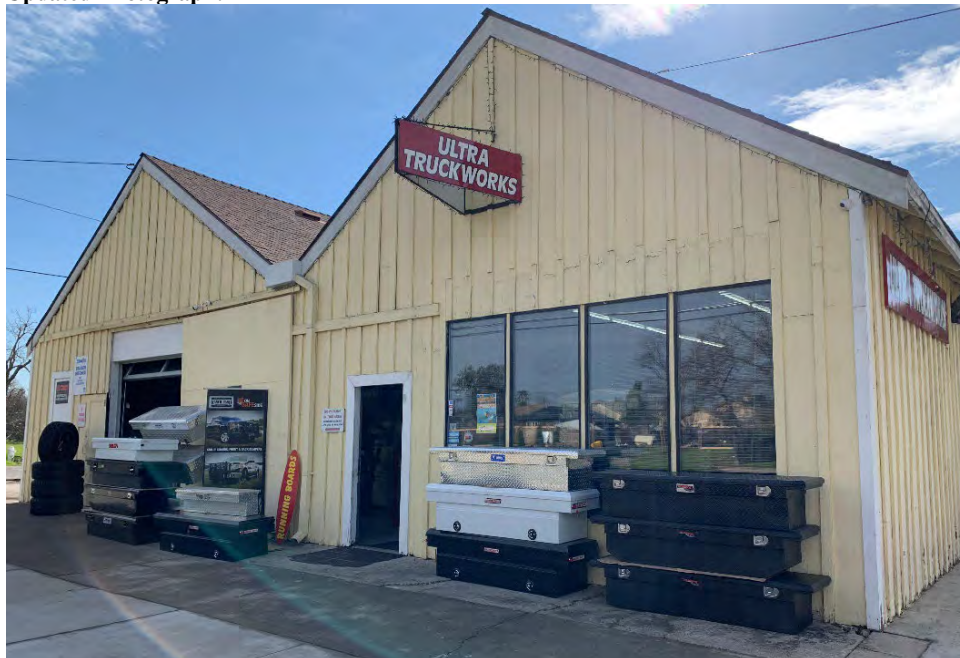
Photograph 1. View southeast of the north and west elevations.
