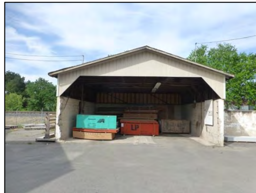
Photograph 10. East elevation of non-contributing storage bldg.
