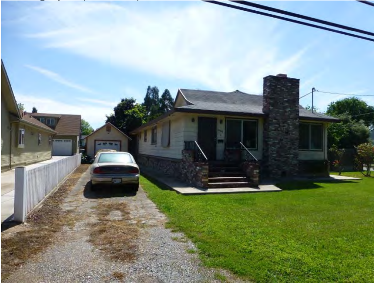
Photograph 2. View southwest of north and east elevations. Detached garage is visible in the background. Taken 4/9/14, #0565.
