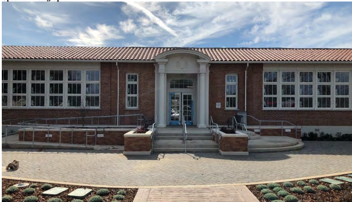
Photograph 1: View south of north elevation.
