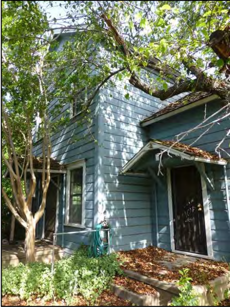
Photograph 3. Front (south) façade. Camera facing northwest.
