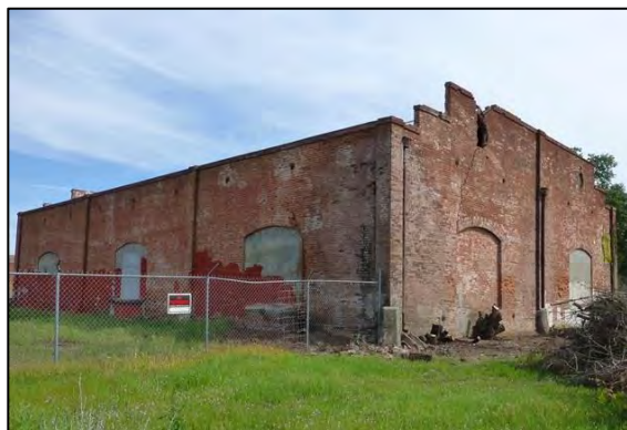
Photograph 14. West & south elevations of Bldg. 2. Camera facing northeast.
