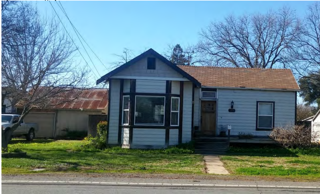
Photograph 1. View northwest of the south and east elevations.
