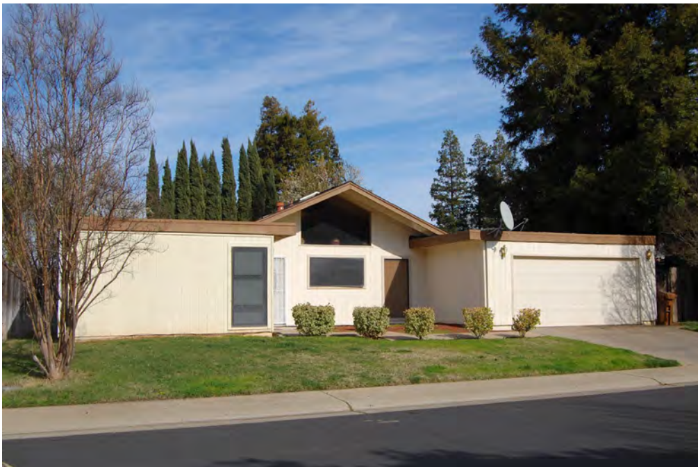
Photograph 3. Representative view of single-family residence located at 8795 Cheer Court. Taken January 24, 2019.
