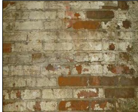
Photograph 12. Structural brick interior wall of the bottling facility of Bldg. 6.
