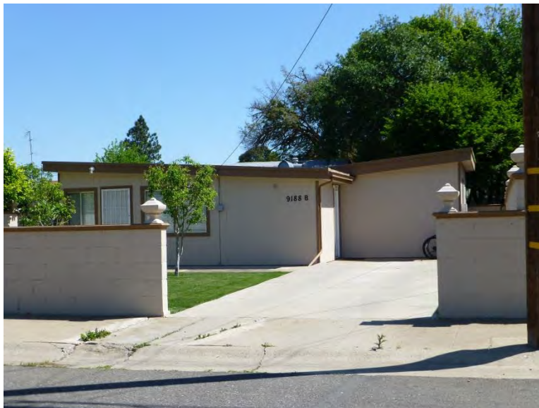
Photograph 3. View northeast and west elevation of second residence (9188 B Grove Street). Taken 4/10/14, #0666.
