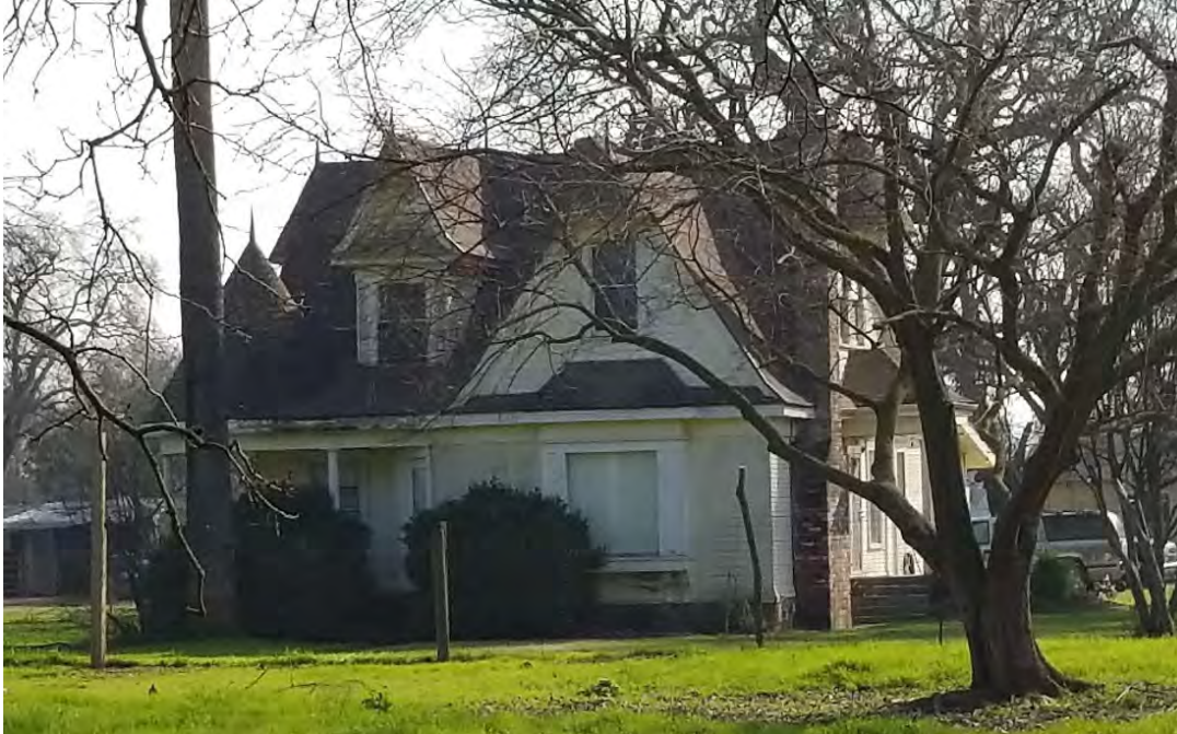
Photograph 1. View southeast of the north and west elevations.
