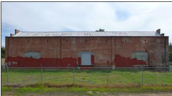
Photograph 2. West elevation. Camera facing east.
