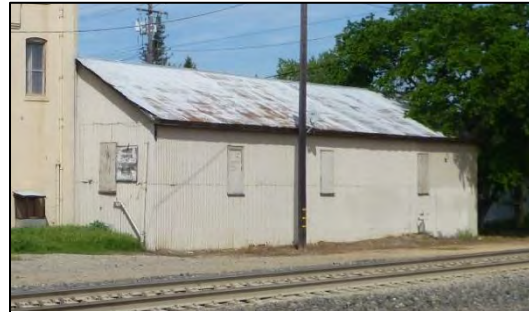
Photograph 3. East and south elevations of the warehouse. Camera facing northwest.
