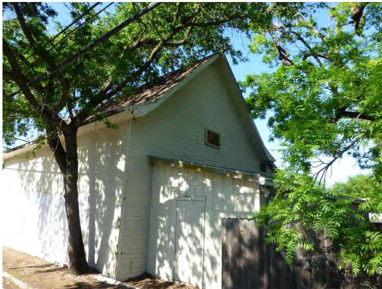
Photograph 2. View southwest of north and east elevation. Taken 4/10/14, #0616.
