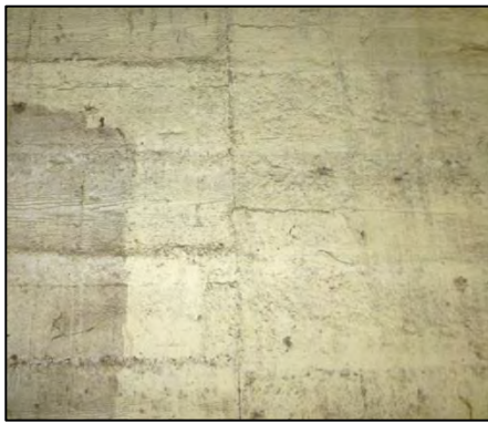
Photograph 11. Board-formed, reinforced concrete interior wall of Bldg. 5.
