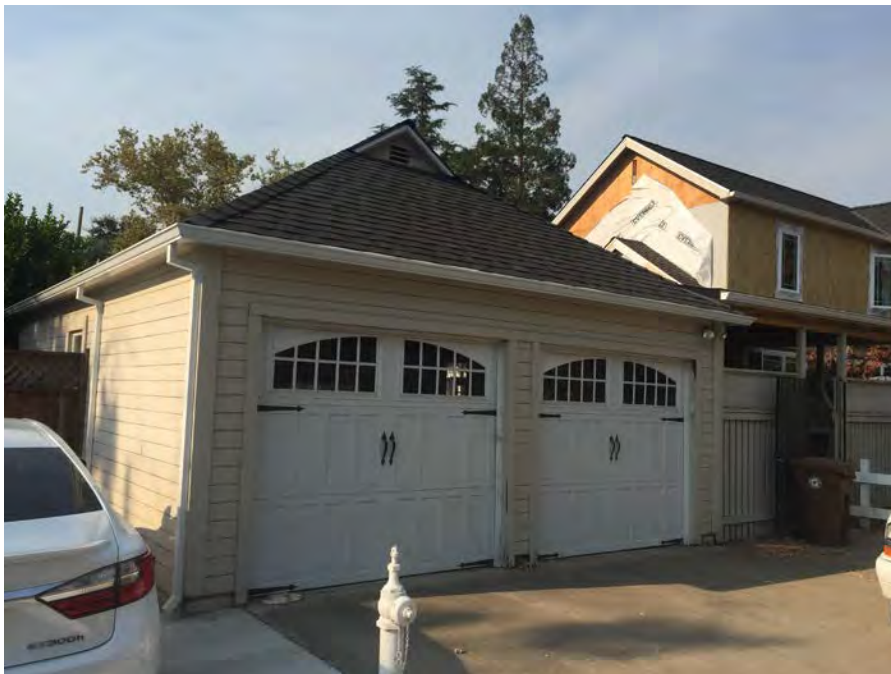
Photograph 5. View southwest of garage depicting replacement garage doors and breezeway addition.
