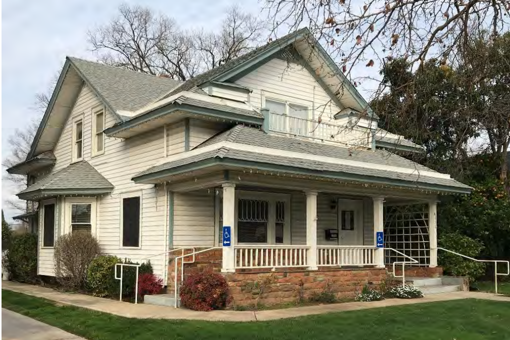
Photograph 1. View northeast of the west and south elevation.
