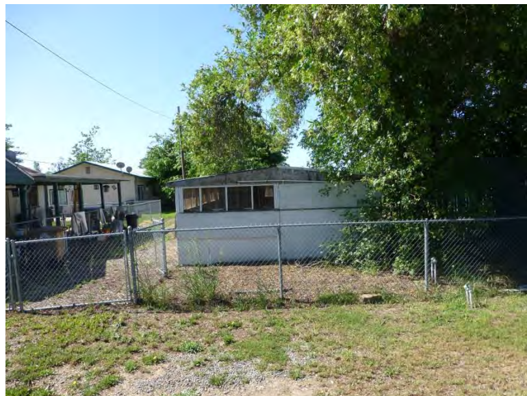
Photograph 2. View southeast of Buildings 1 and 3. Taken 5/11/14.
