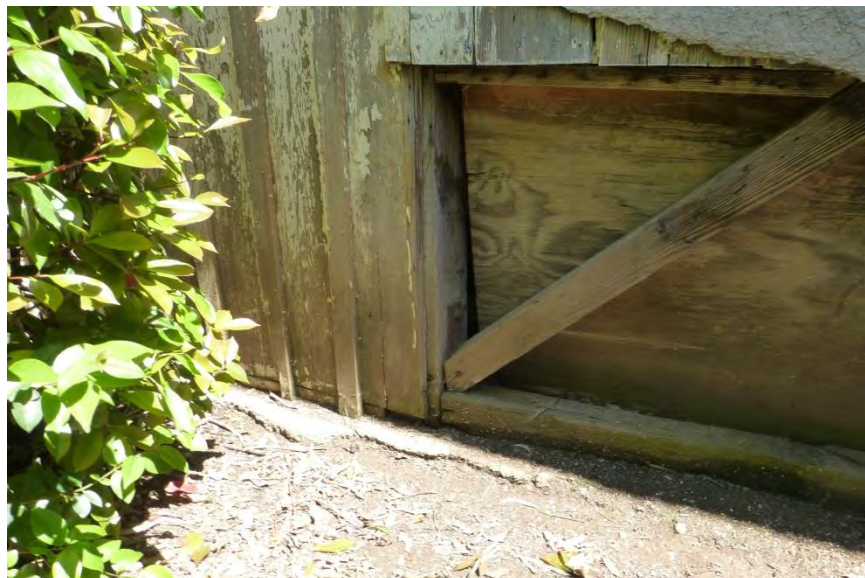
Photograph 2. View northeast of foundation, frame, and wall cladding; taken 4/9/14, #0559.
