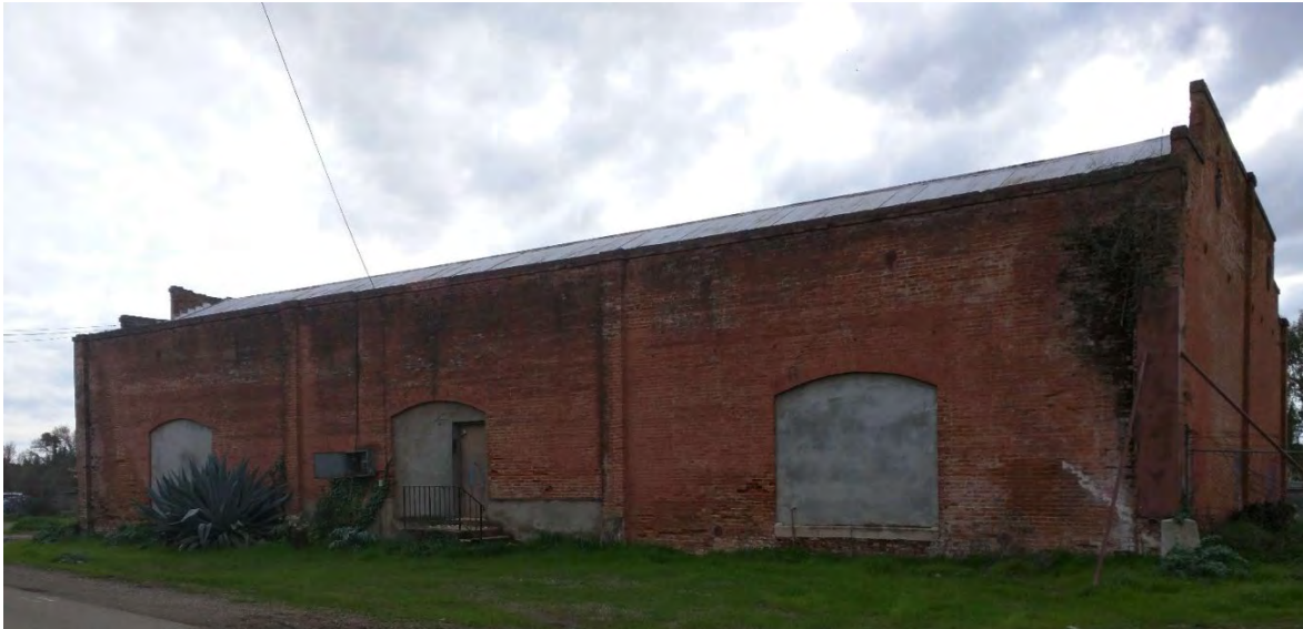
Photograph 1. View southwest of the east and north elevations.
