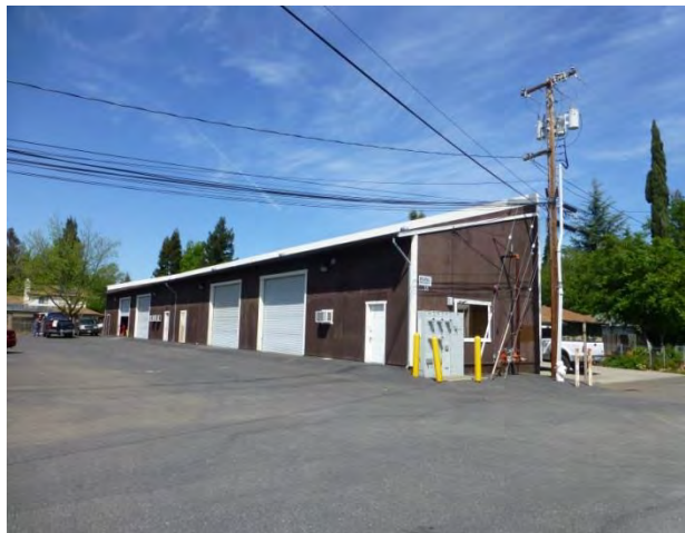
Photograph 3. Building C. View northeast. Taken 4/9/14.
