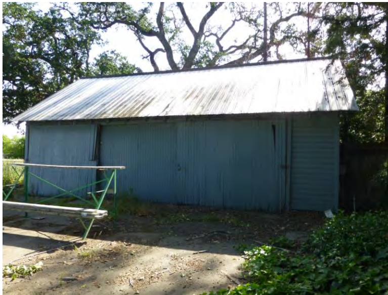
Photograph 2. South elevation of garage. Camera facing northwest. Photo taken May 2, 2014.
