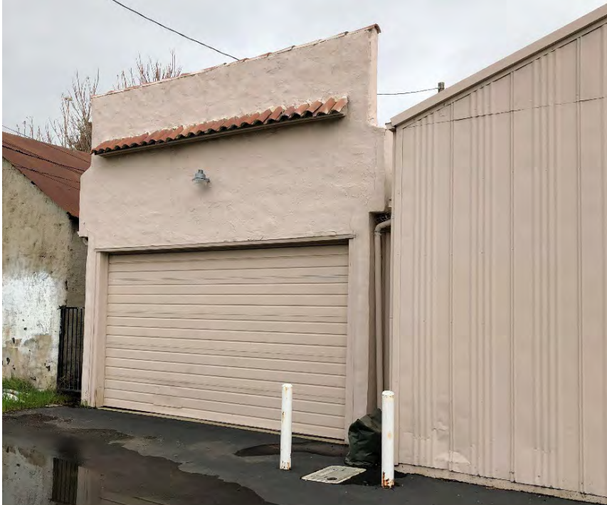
Photograph 1: View northwest of south elevation.
