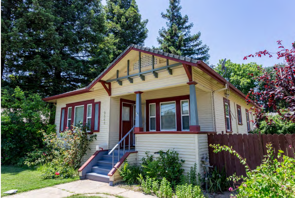
Photograph 1. View northwest of the east and south elevations.
