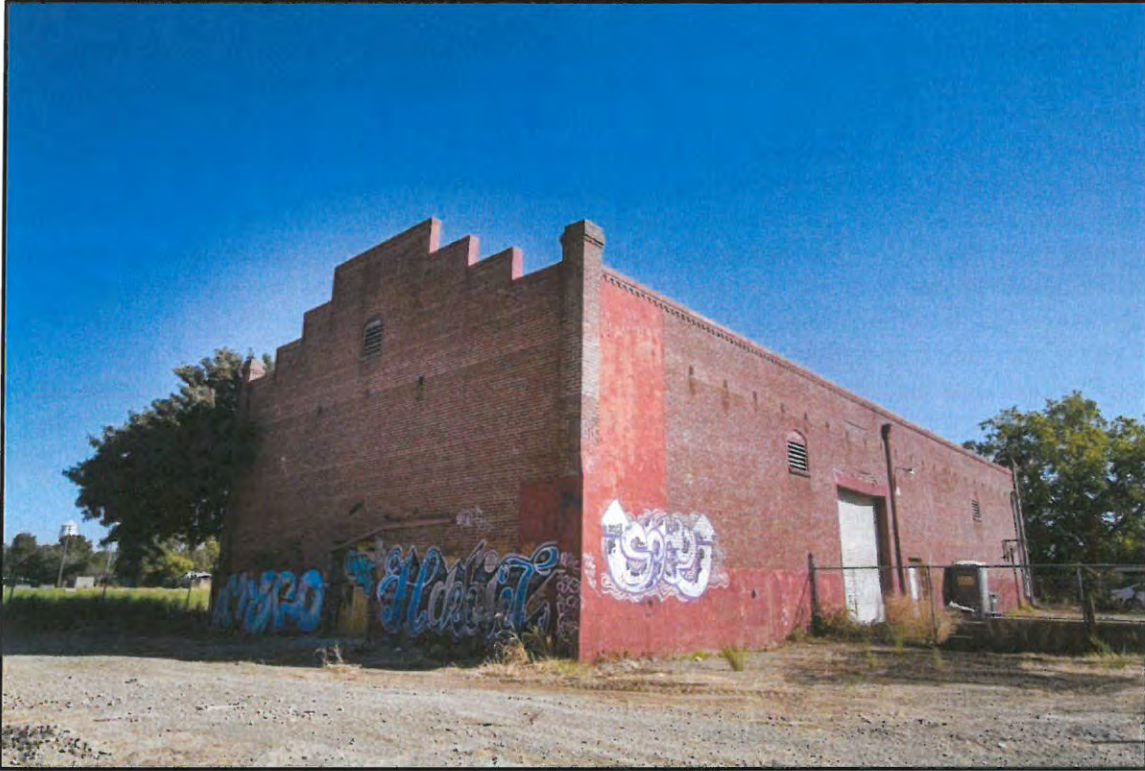
West (rear) and south elevations, view to the northeast.
