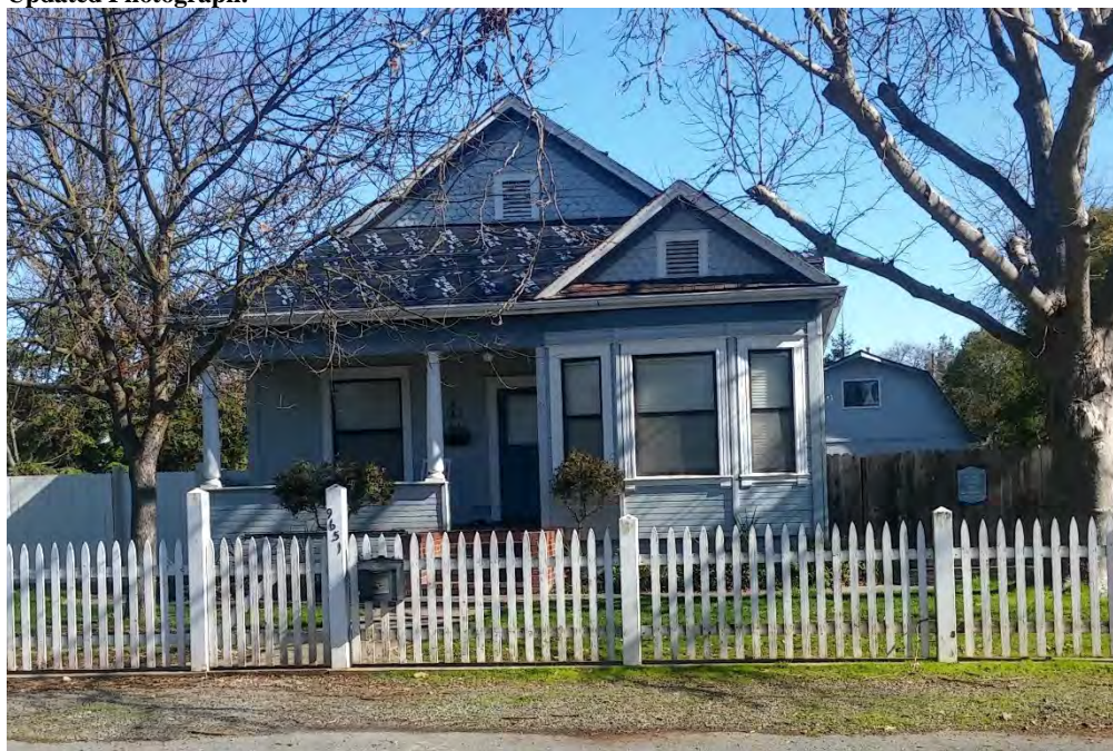
Photograph 1. View east of west façade.
