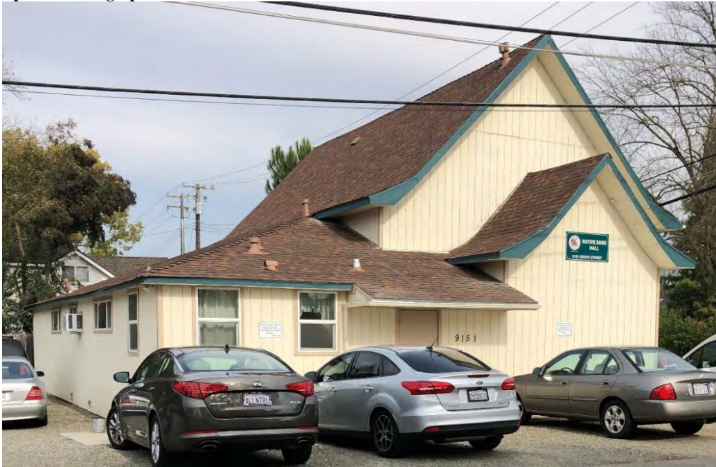
Photograph 1. View northeast of the west and south elevations.
