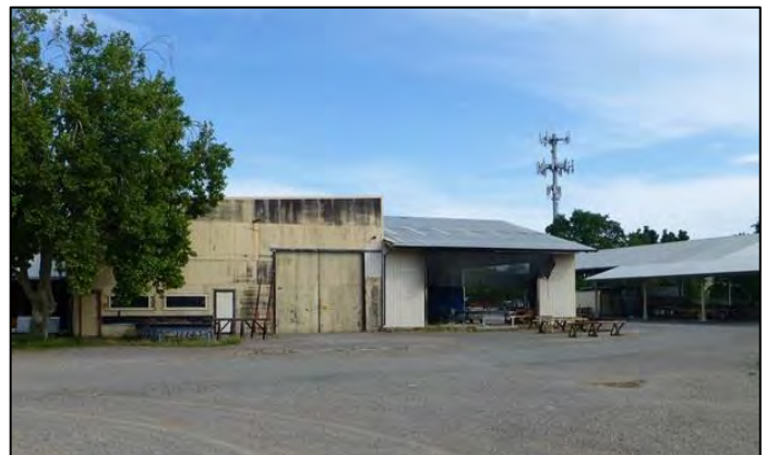
Photograph 4. At the left and center are two later additions affixed to the south end of the original 1915 facility housing the sherry oven. The gable roof pole barn at the right is a non-contributor to the district built in 1976.
