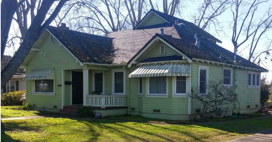
Photograph 1. View southwest of east and north elevations.
