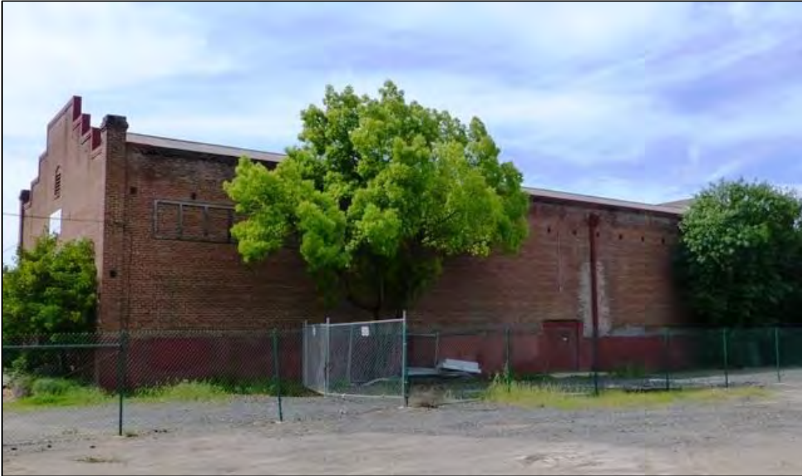
Photograph 4. North and east elevations of Elk Grove Winery Warehouse. Camera facing southwest.
