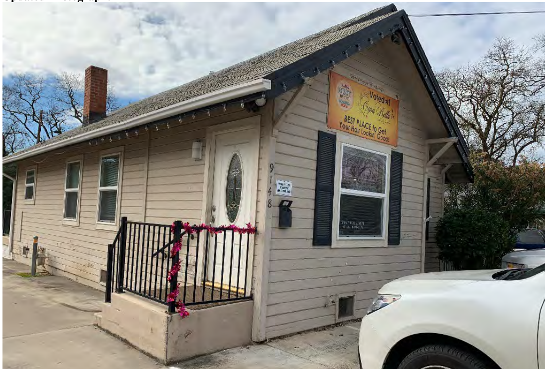
Photograph 1. View southwest of the north and east elevations.
