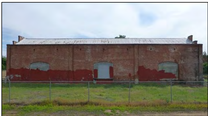
Photograph 15. West elevation of Bldg. 2. Camera facing east.
