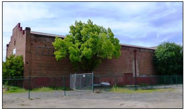
Figure 5. Elk Grove Winery Warehouse, built circa 1900. North & east elevations. Camera facing south.
