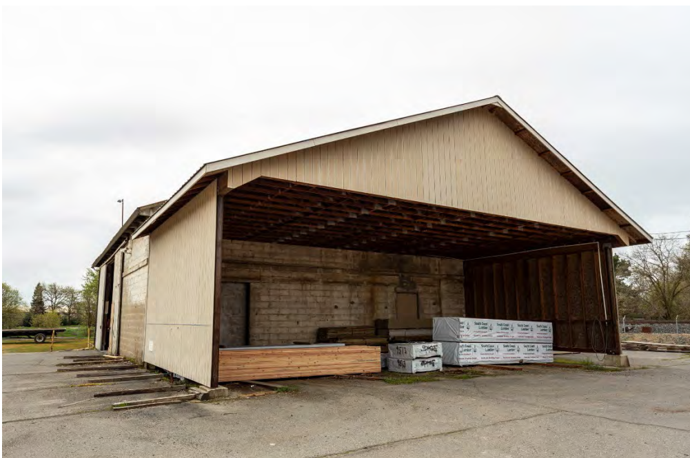
Photograph 2. View southwest of the east and north elevations of Building 3.
