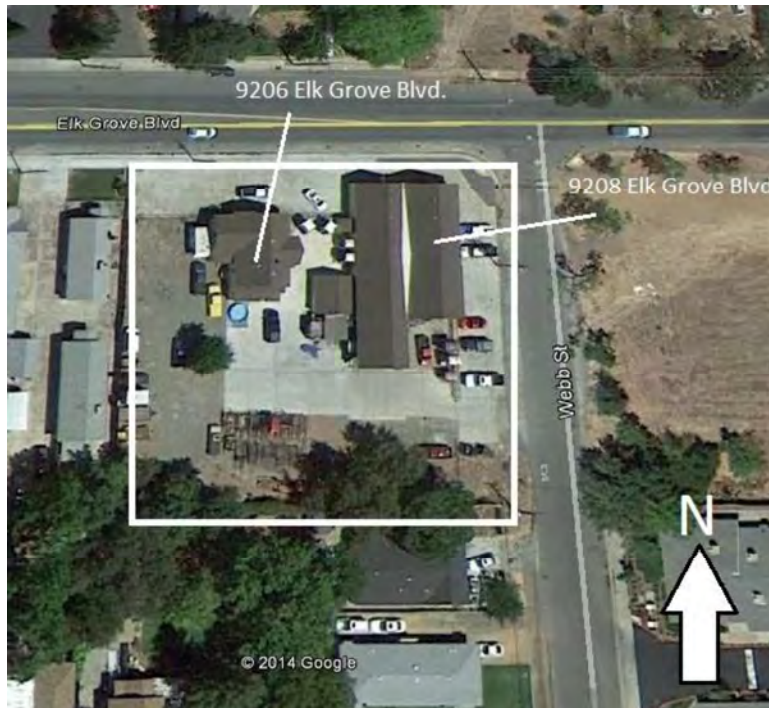
Figure 1. Blacksmith Shop at 9208 Elk Grove Boulevard, which shares a parcel with the Percy Webb Residence at 9206 Elk Grove Boulevard.
