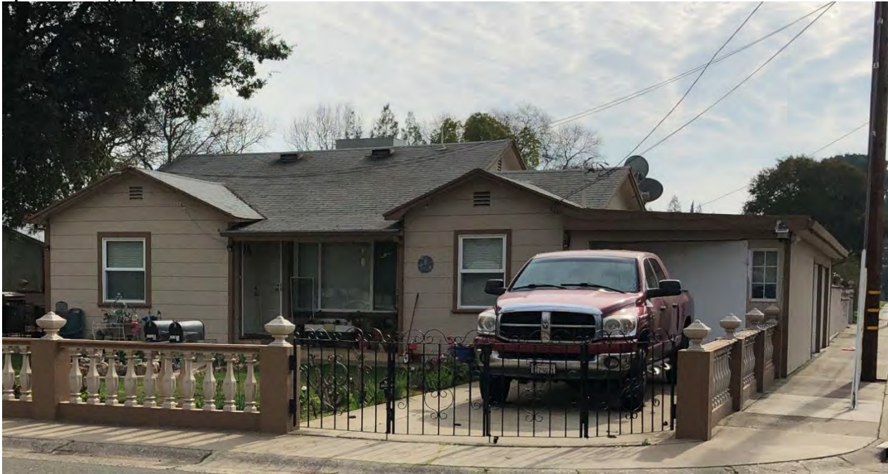
Photograph 1. View southeast of the north elevation.
