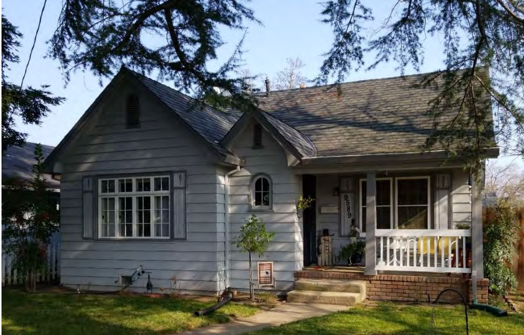
Photograph 1. View northeast of west elevation.
