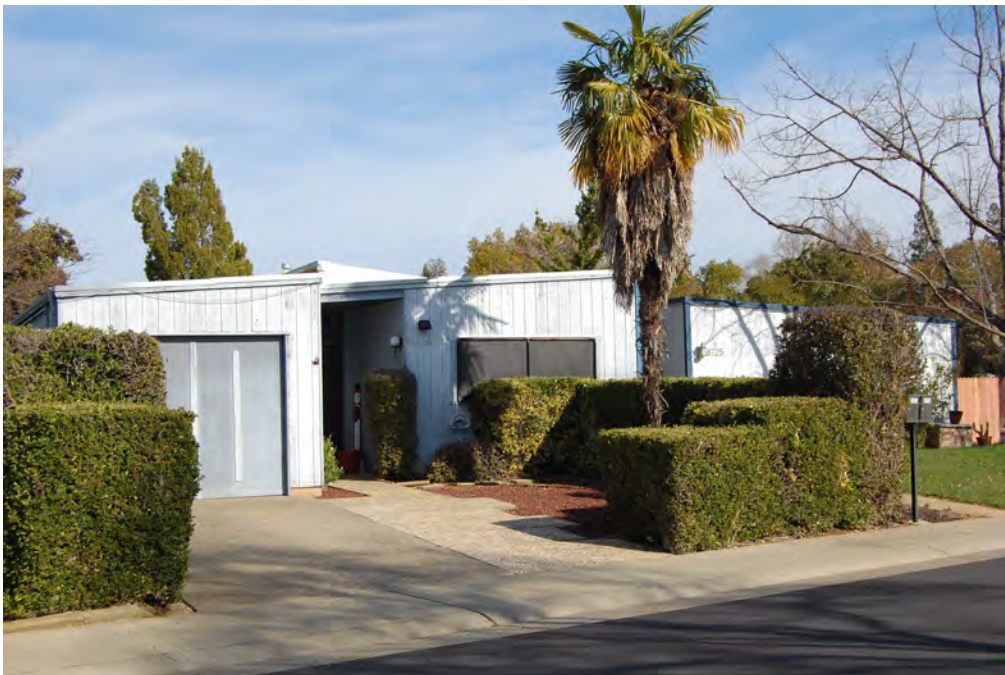
Photograph 5. Representative view of multi-family residence located at 8721 Seckle Court. Taken January 24, 2019.
