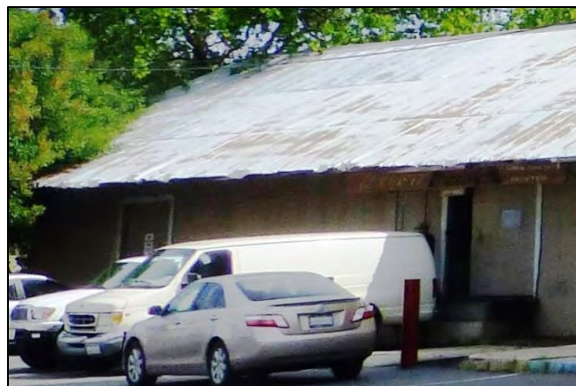
Photograph 6. West elevation of the warehouse. Camera facing east.
