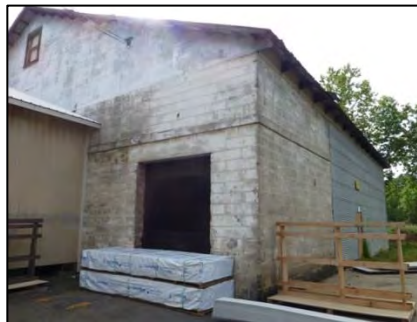
Figure 11. Bldg. 4-Winery Warehouse.
