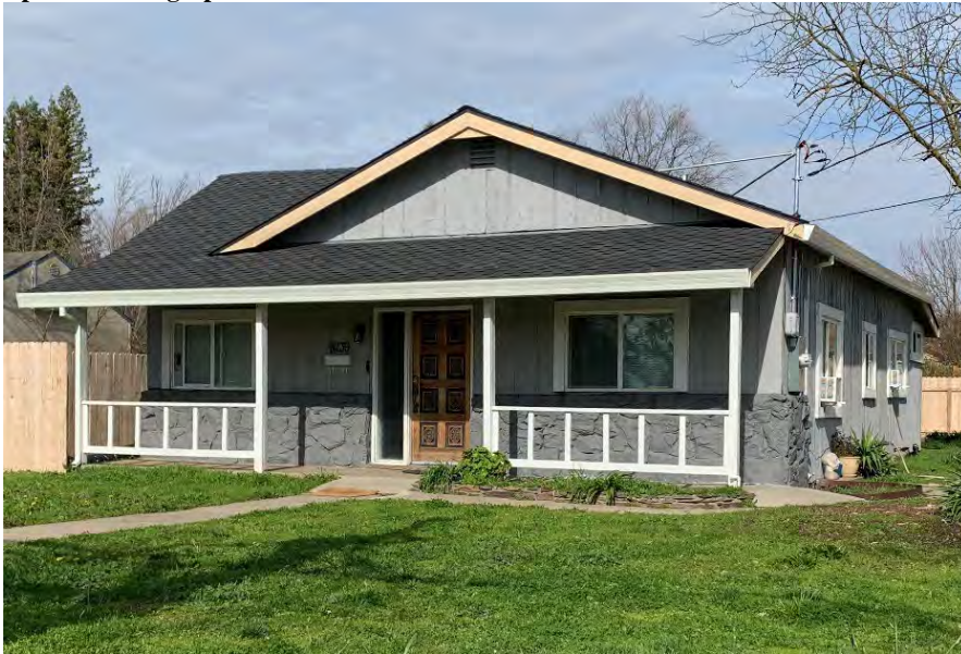
Photograph 1: View northwest of the south and east elevation of Residence 1.
