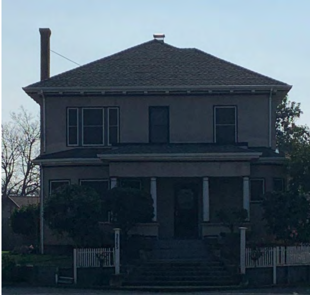
Photograph 1. View southwest of the east elevation.
