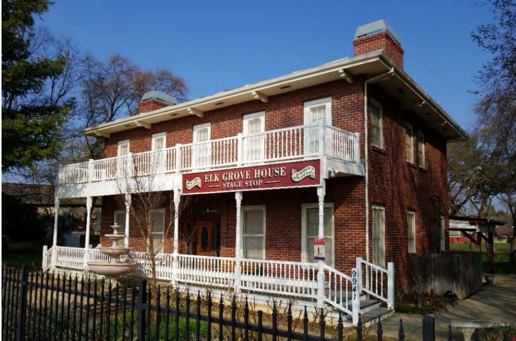
Photograph 1. View north of southwest and southeast elevations.
