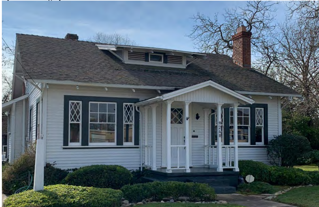
Photograph 1. View southwest of the north and east elevations.
