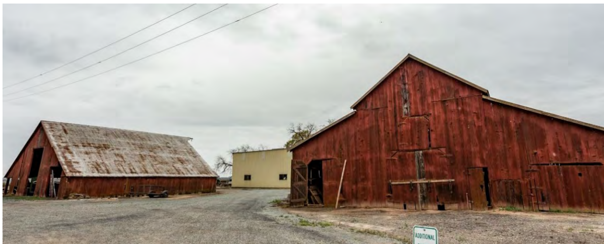
Photograph 2. View southwest of Barn 2, Ancillary Building 2, and Barn 1.
