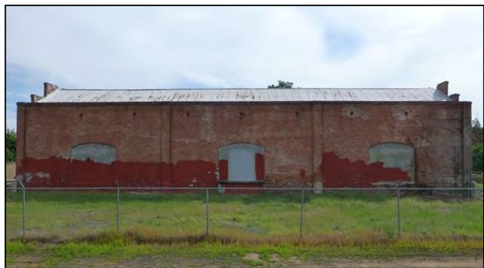
Photograph 15. West elevation of Bldg. 2. Camera facing east.
