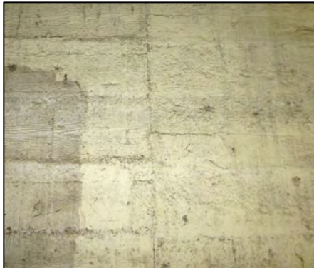
Photograph 7. Board-formed, reinforced concrete interior wall of Bldg. 5.
