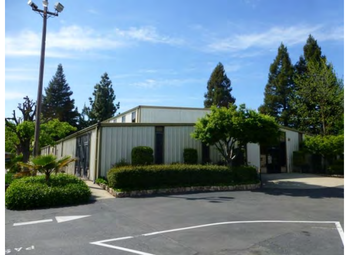
Photograph 5. View northwest of church offices.
