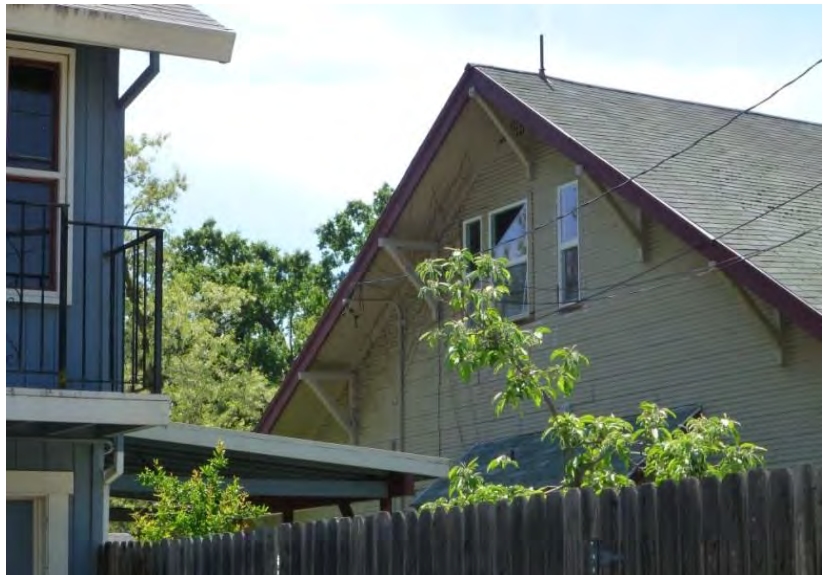
Photograph 2. View southwest of east elevation. Taken 4/9/14, #0561.
