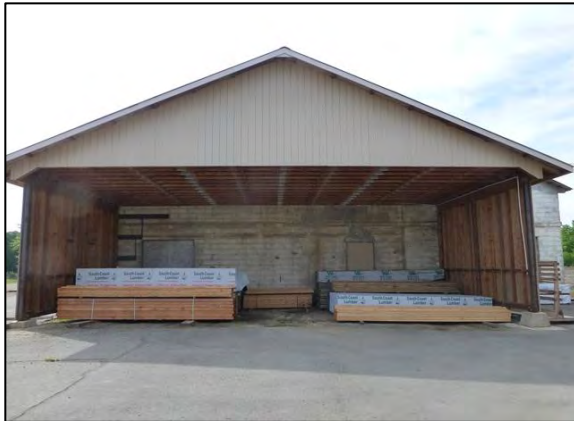
Photograph 13. North elevation of Bldg. 4 with an affixed 1984 addition. Camera facing south.
