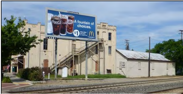
Photograph 2. Overview of warehouse (right) & IOOF Hall (left). Camera facing northwest.
