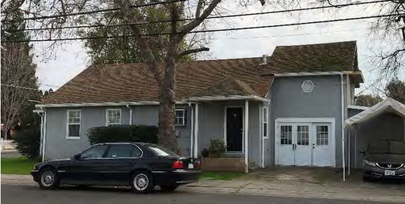
Photograph 1: View south of north elevation.
