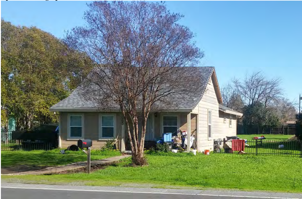
Photograph 1. View northeast of west and south elevations.
