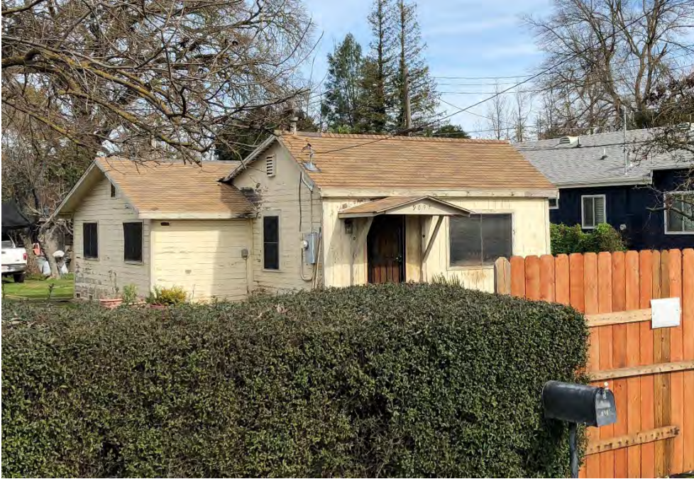
Photograph 1. View northeast of the west and south elevations.
