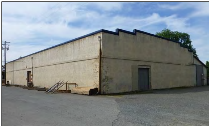
Photograph 16. North & east elevations of Bldg. 5. The original concrete block exterior walls of this building have been altered with a layer of stucco .
