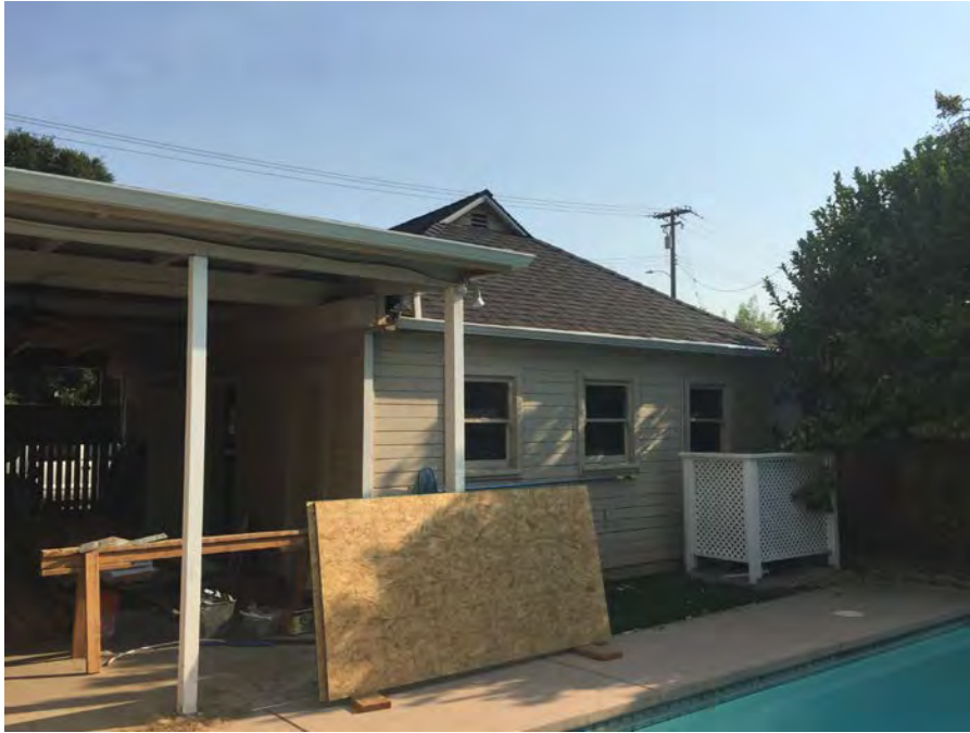
Photograph 6. View northeast of garage.
