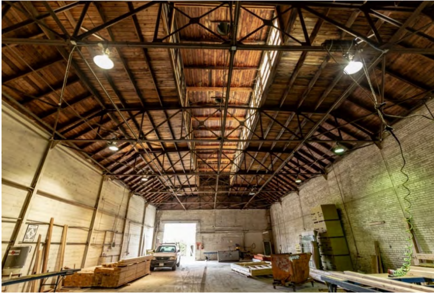
Photograph 1. View northwest of Elk Grove Vineyard Association Winery Building 6 interior.
