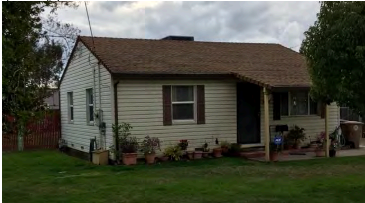
Photograph 1. View southwest of the east and north elevations.
