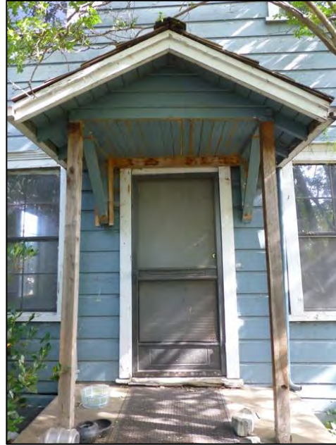
Photograph 4. Original main entry on south façade. Camera facing north.
