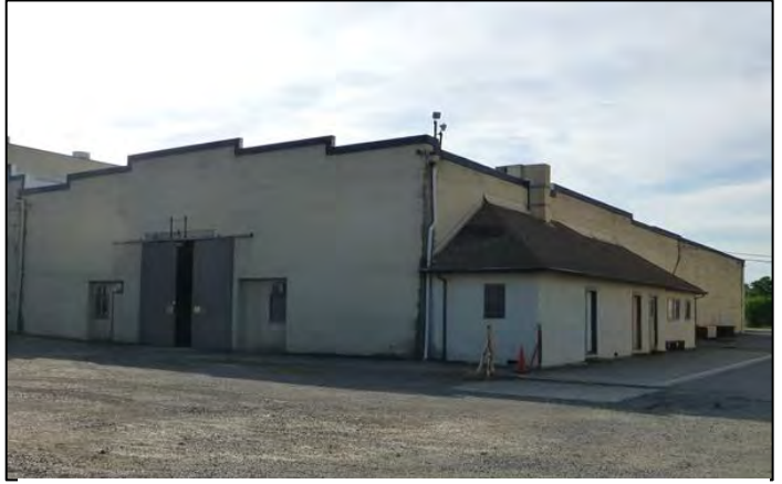
Photograph 3. North and west elevations of Bldg. 5. The half-hipped, truck-scale office appended to the west elevation is not an original feature of the building as constructed in 1915.
