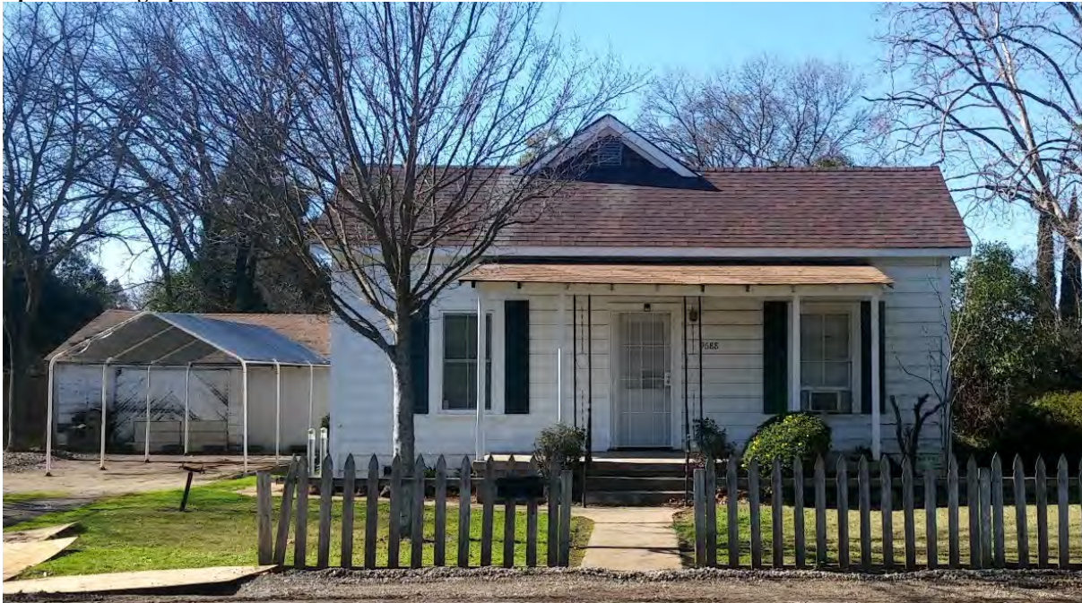
Photograph 1. View west of east facade.
