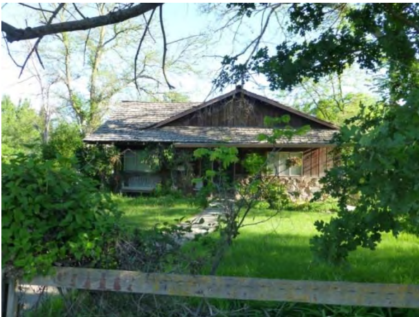
Photograph 5. South elevation of Residence 1. Camera facing north.
