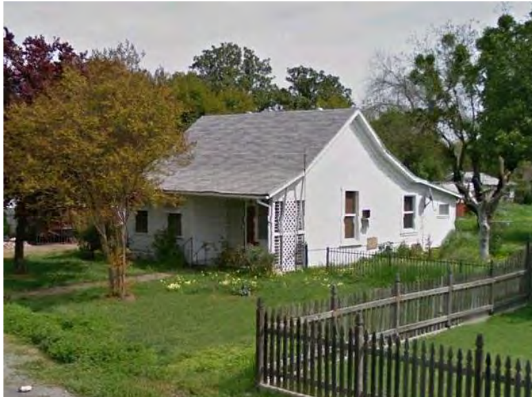
Photograph 3. View northeast of residence. Note the original roofline.
