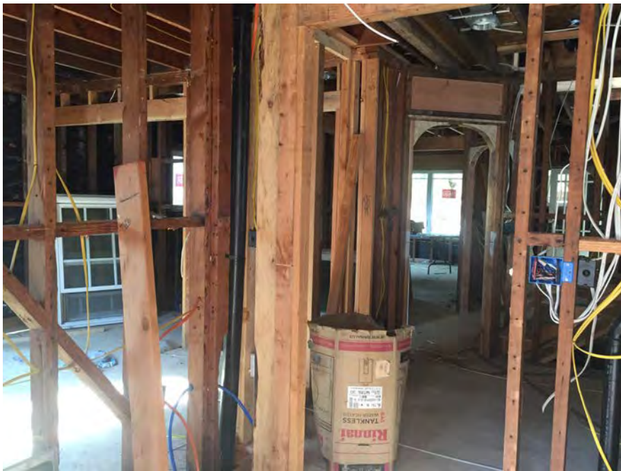
Photograph 7. Interior view of residence depicting the breadth of renovation.
