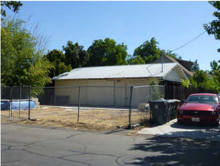
Photograph 3. View northeast of workshop. Taken 5/11/14, # 0019.
