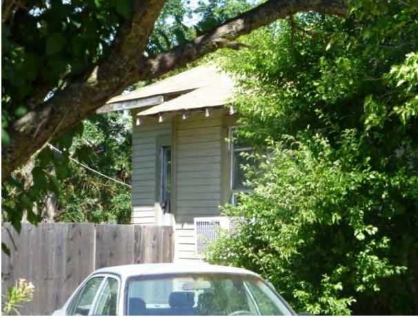
Photograph 3. South elevation of Gage Residence. Camera facing northwest.
