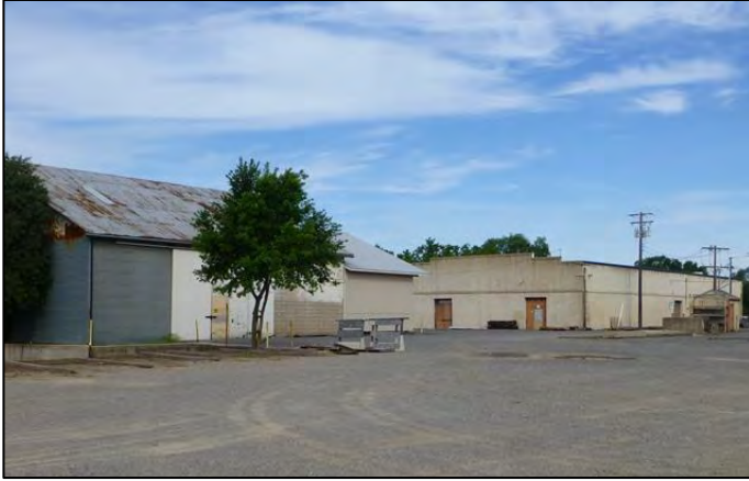
Photograph 11. Overview showing the two surviving 1909 EGVA winery buildings designed by the firm of Toulouse & Delorieux. Bldg. 4 (left) and Bldg. 3 (right). Camera facing northwest.
