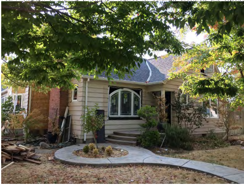
P5a. Photograph or Drawing (Photograph required for buildings, structures, and objects.)
