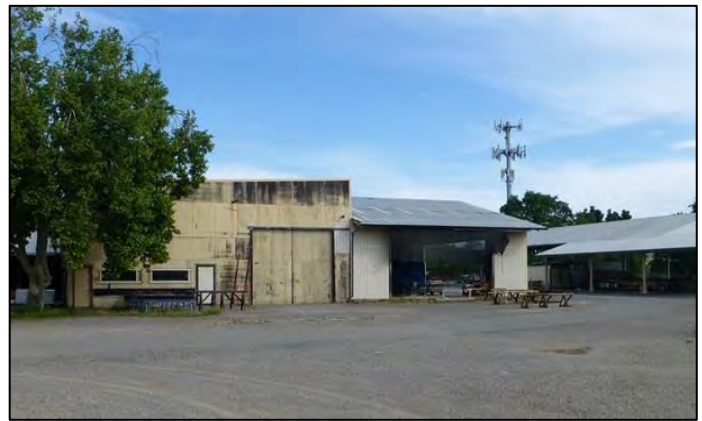
Photograph 5. At the left and center are two later additions affixed to the south end of the original 1915 facility housing the sherry oven. The gable roof pole barn at the right is a non-contributor to the district built in 1976.
