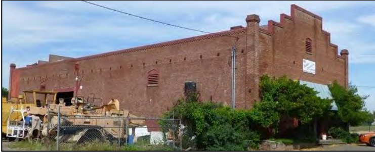
Photograph 16. South & east elevations of Bldg. 1. Camera facing northwest.
