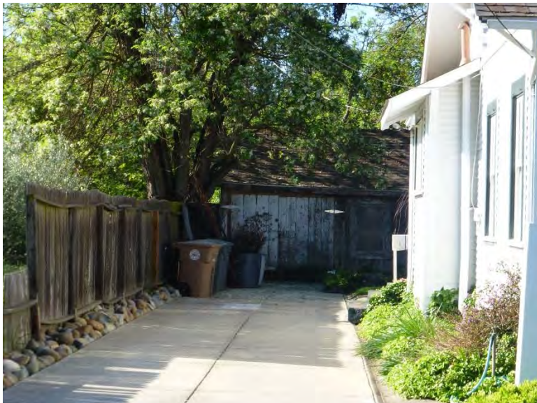
Photograph 2. View south of detached garage, north elevation. Taken 4/10/14, #0609.
