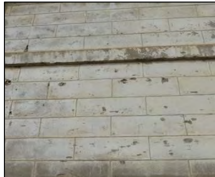
Photograph 18. Bldg. 4-Section of concrete-block wall.
