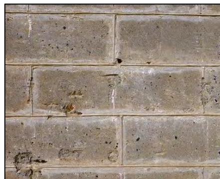
Photograph 19. Bldg. 4-Closeup of original concrete block wall.
