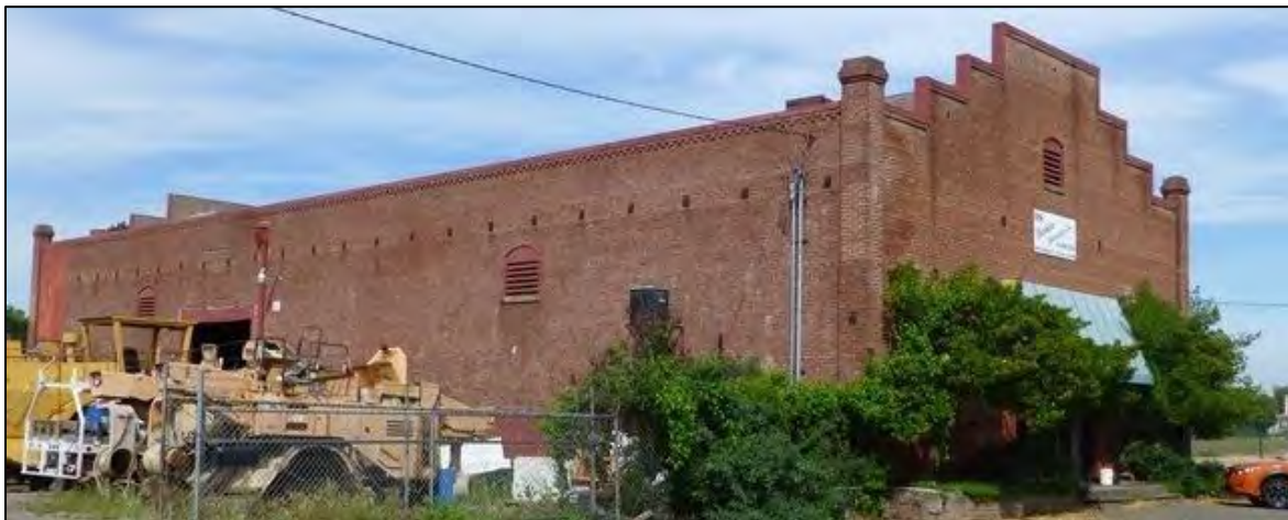
Photograph 3. South and east elevations of Elk Grove Winery Warehouse. Camera facing northwest.
