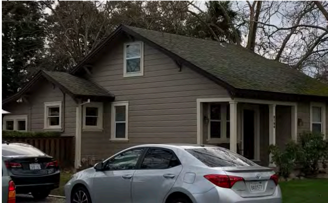
Photograph 1. View southwest of the east and north elevations.
