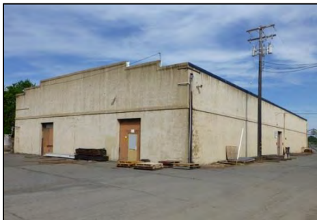
Figure 10. Bldg. 3-Fermenting & Wine Storage Facility.
