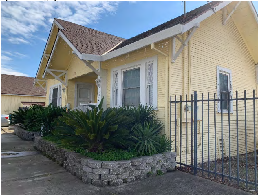
Photograph 1. View southwest of the north and east elevations.
