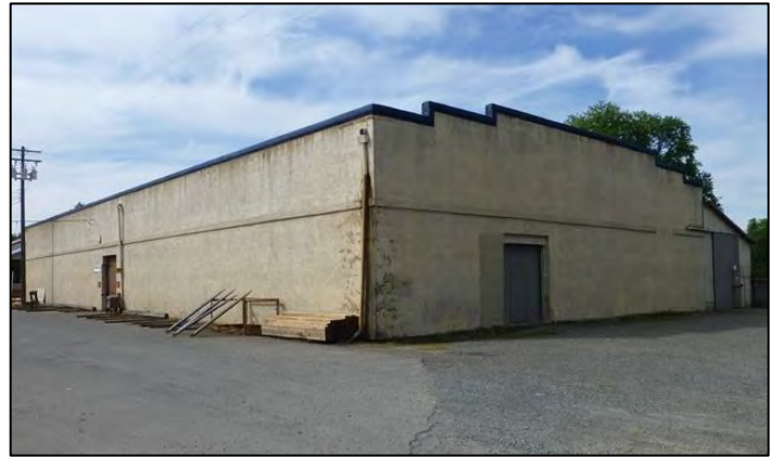
Photograph 13. North & east elevations of Bldg. 5. The original concrete block exterior walls of this building have been altered with a layer of stucco .
