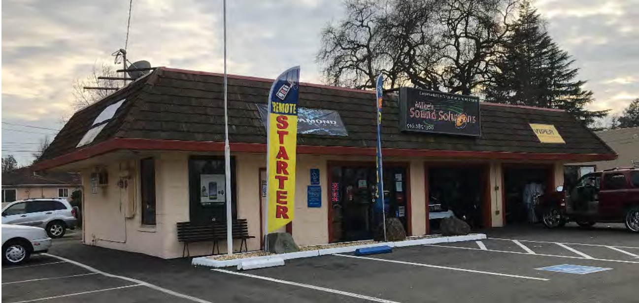
Photograph 1: View southwest of east and north elevations.
