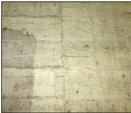
Photograph 11. Board-formed, reinforced concrete interior wall of Bldg. 5.
