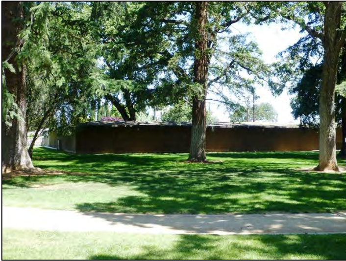
Photograph 8. View northeast of non-contributing maintenance facility/office complex (#8). Park officials made an attempt to screen its presence with the brown fencing.
