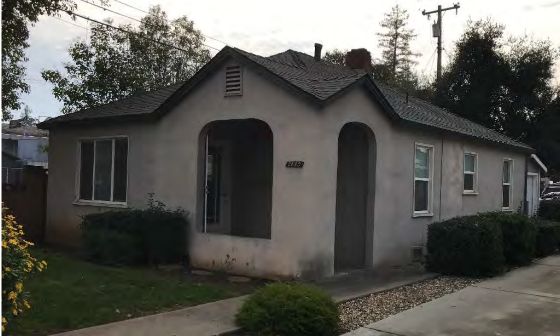
Photograph 1: View southwest of east and north elevations.
