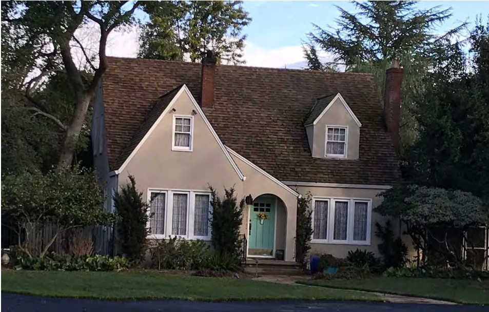
Photograph 1. View east of the west elevation.
