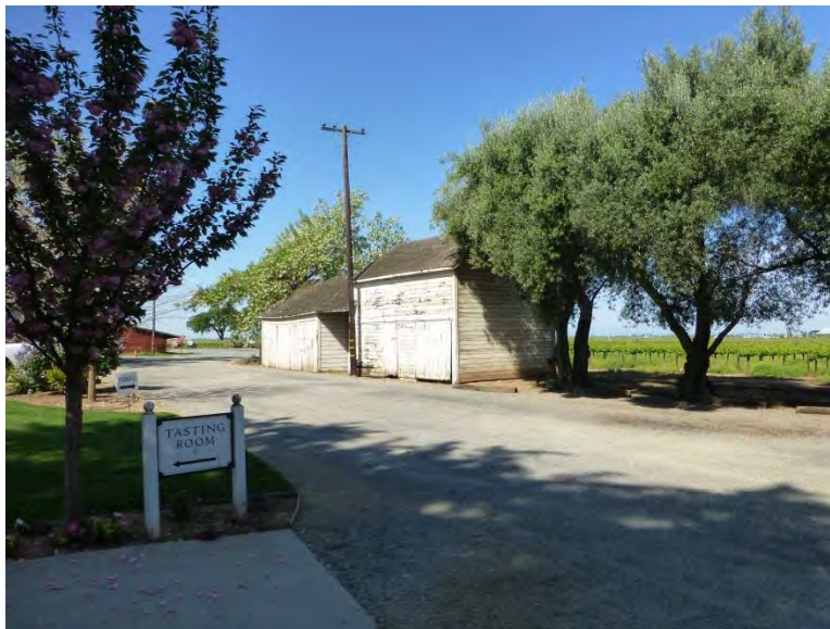
Photograph 3. View northwest of ancillary building. Taken 4/9/14, #0533.
