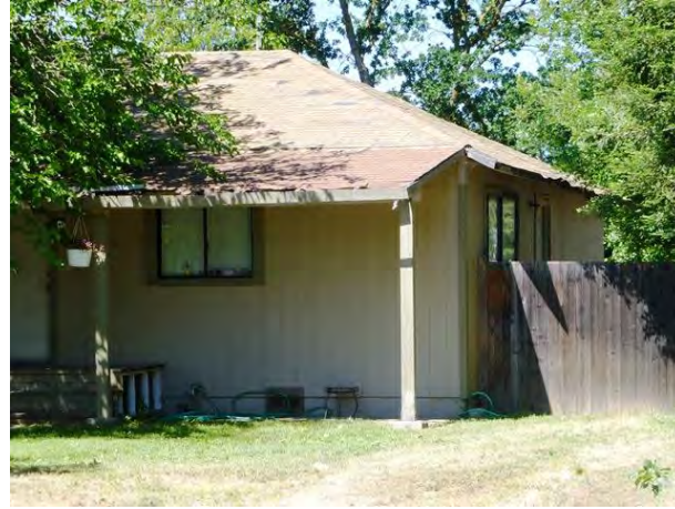
Photograph 4. East & north elevations of Gage Residence. Camera facing southwest.
