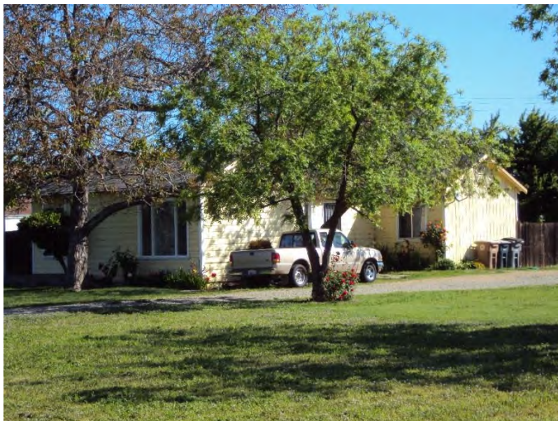
Photograph 2. Residence 2, south and west elevations. Camera facing northeast. Taken April 10, 2014.
