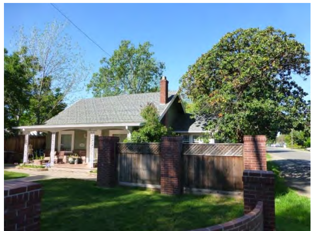
Photograph 2. View southwest of east elevation. Taken 4/10/14
