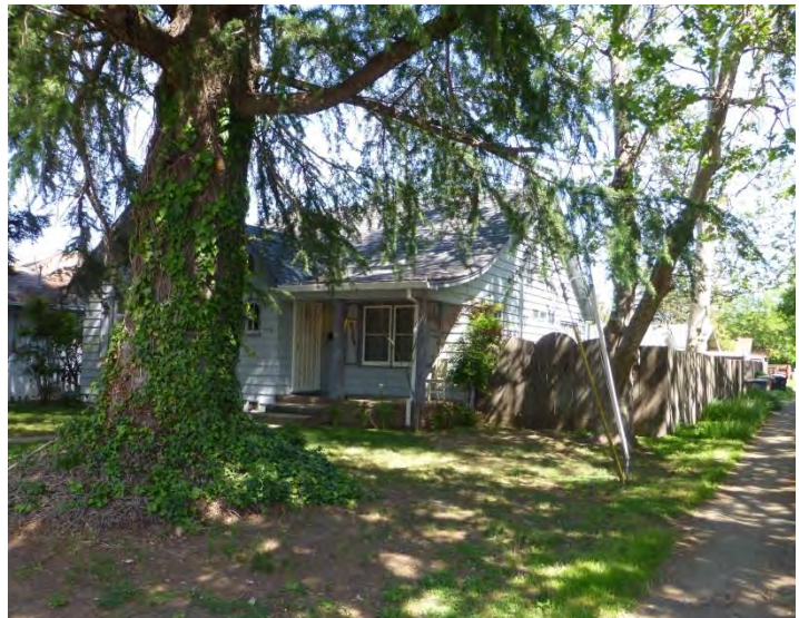
Photograph 2. View northeast of south and west elevations.
