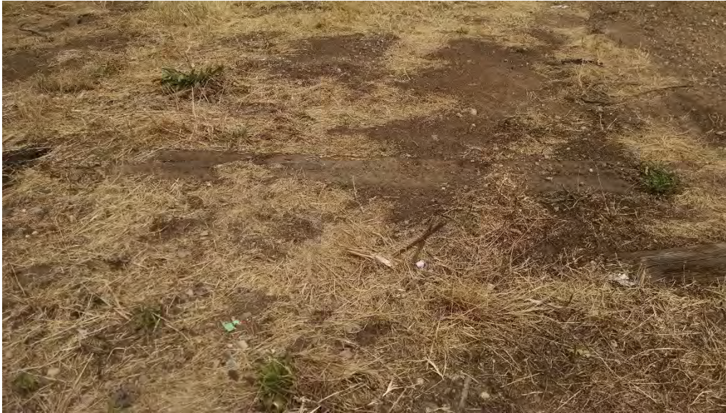
Photo 2. View north of buried wood tie.
