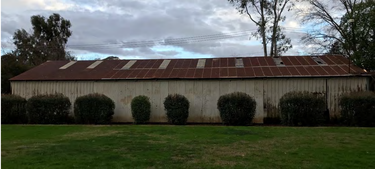
Photograph 1. View east of the west elevation.
