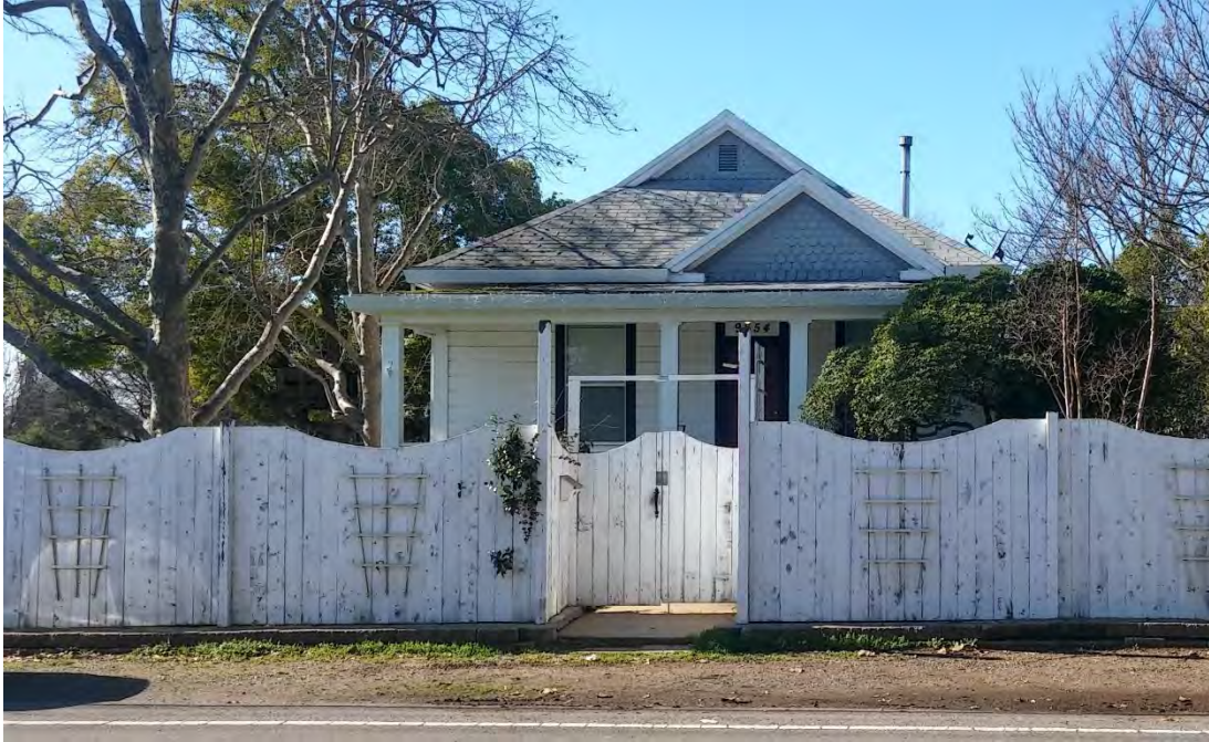
Photograph 1. View west of east façade.
