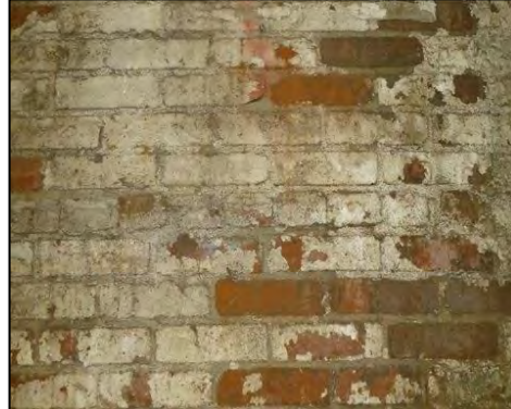
Photograph 8. Structural brick interior wall of the bottling facility of Bldg. 6.
