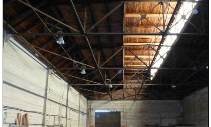
Photograph 6. Bldg. 6, by contrast, displays a steel-truss roof system and no interior posts due to the narrower width of the building.
