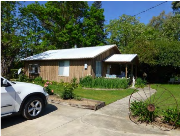
Photograph 4. View northwest of Office Building 1.
