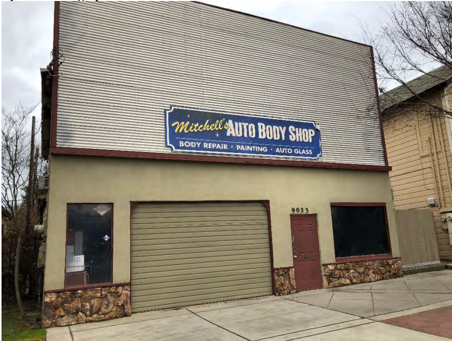
Photograph 1: View north of south elevation.
