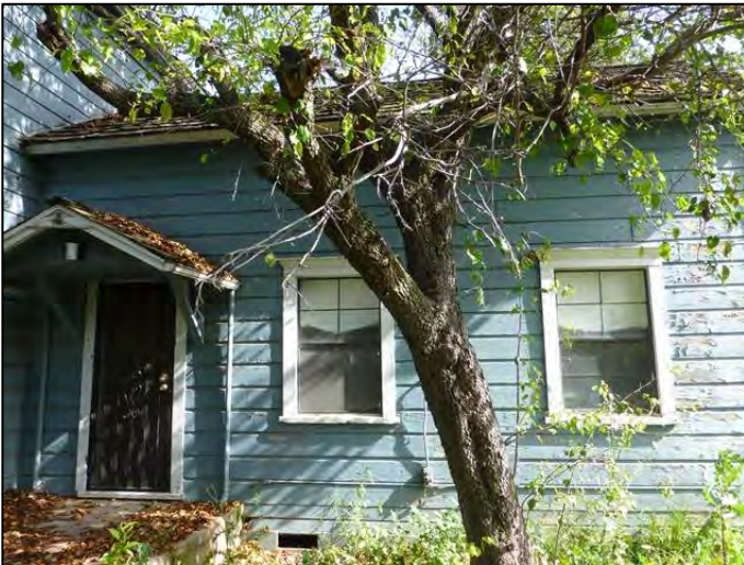
Photograph 5. South façade of the addition appended to east elevation of the original two-story massing. Camera facing north.
