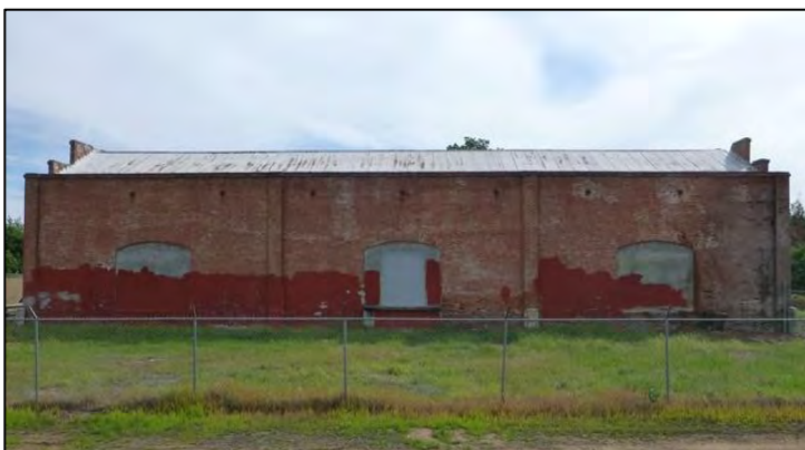
Photograph 2. West elevation. Camera facing east.
