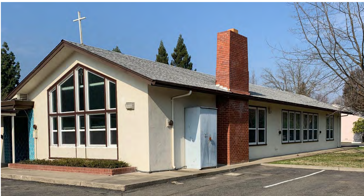
Photograph 2. View northwest of the south and east elevations of the education building.
