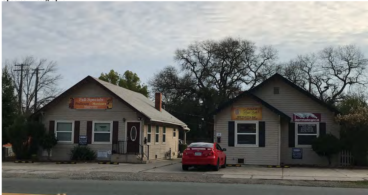
Photograph 1. View southeast of the north and west elevations.
