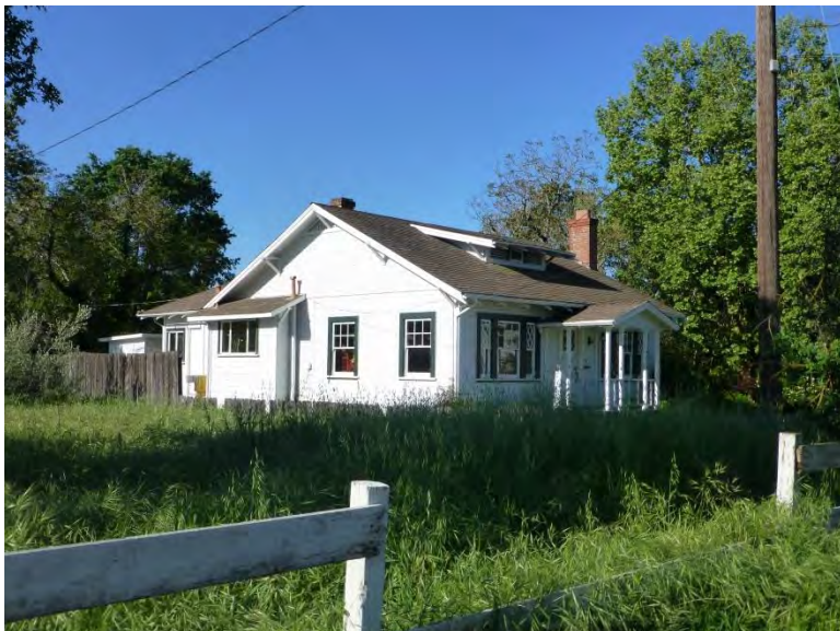
Photograph 3. View southwest of north and east elevations. Taken 4/10/14, #0606.
