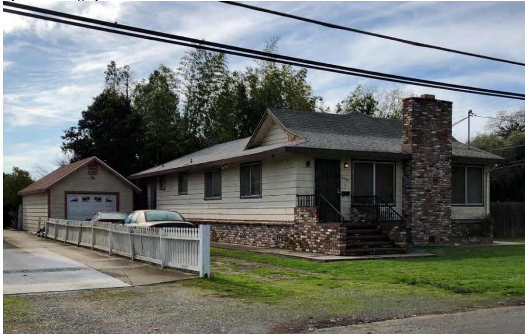
Photograph 1. View southwest of the east and north elevations.
