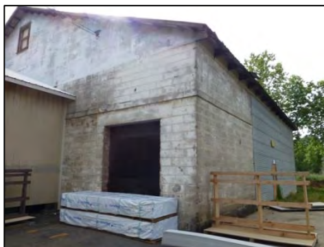
Photograph 17. Bldg. 4-north & west elevations of winery warehouse.
