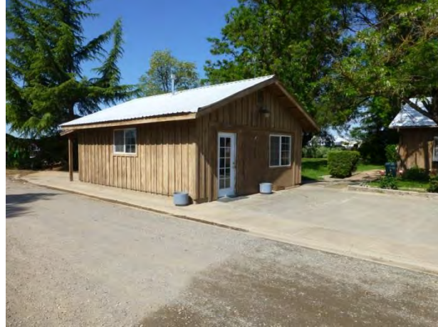
Photograph 3. View northwest of Office Building 2.
