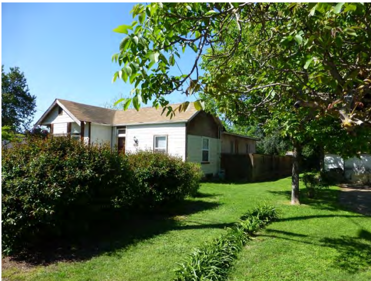
Photograph 2. View southwest of north and east elevations. Note the large flat-roofed room addition in the northwest corner. Taken 4/10/14, #0646.
