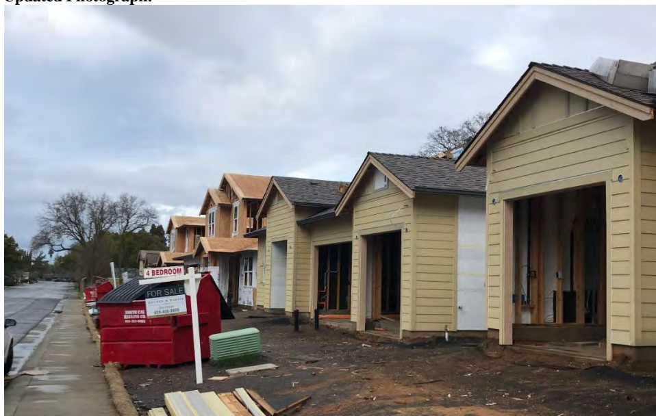
Photograph 1. View of new construction at the former Hunt Family Residence location.
