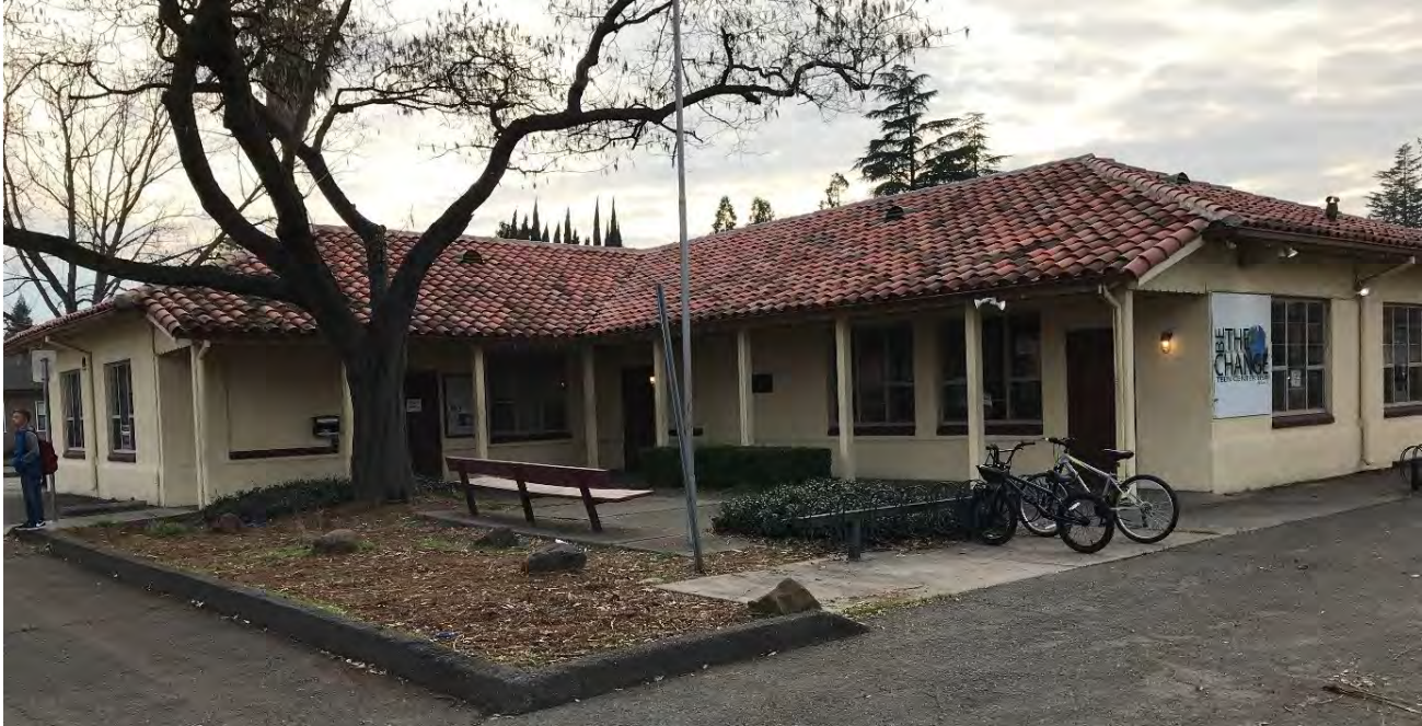
Photograph 1: View southwest of east and north elevations.
