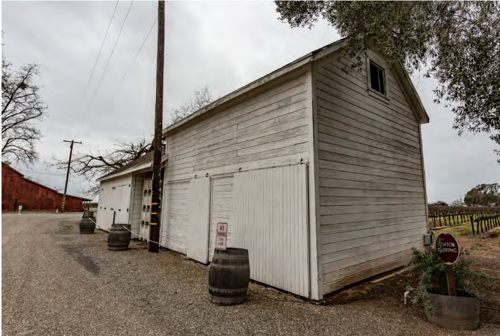
Photograph 3. View west of the southeast and northeast elevations of Ancillary Building 1.
