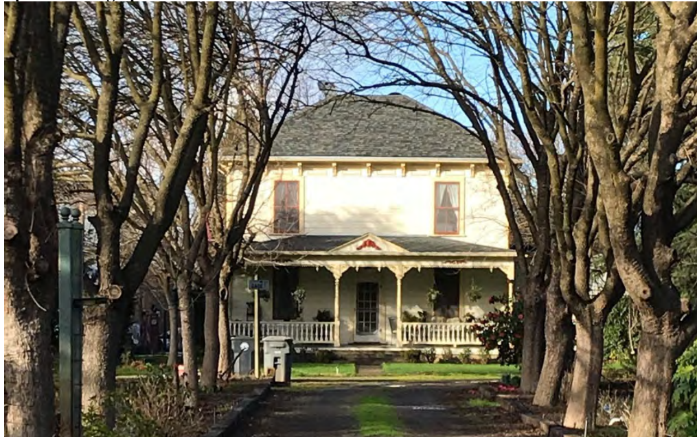
Photograph 1. View north of south elevation.
