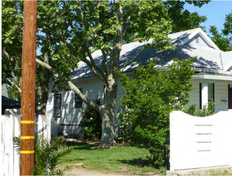
Photograph 2. View facing northwest of south and east elevations. Taken 4/10/14, #0634.
