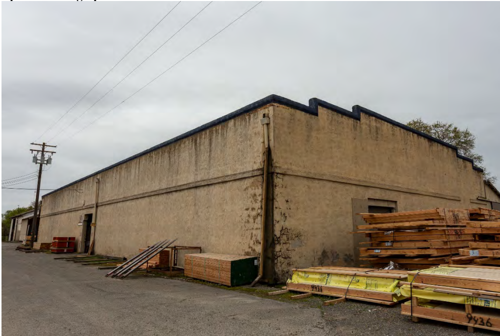
Photograph 1. View southwest of the east and north elevations of Building 3.
