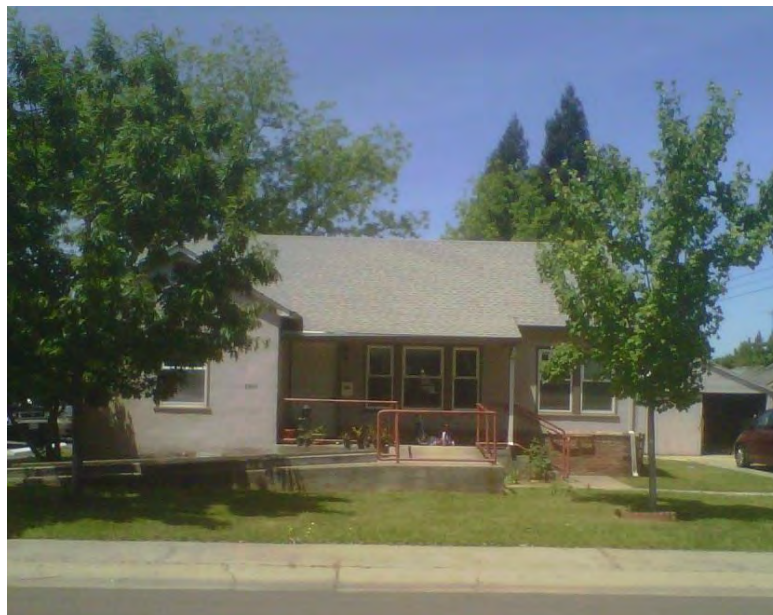
Photograph 6. View west of residence and detached garage at 9540 Batey Avenue.
