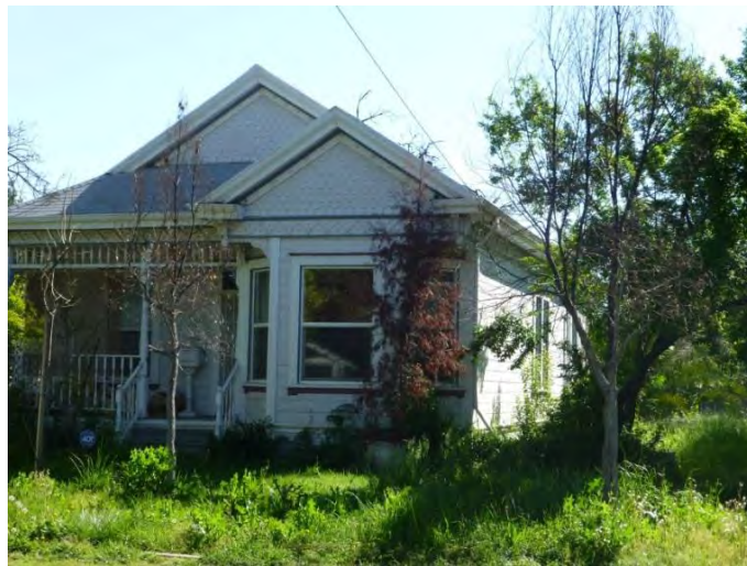
Photograph 2. View facing northeast of south and west elevations of Everson/Heart Residence.
