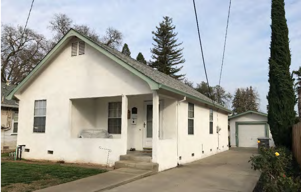
Photograph 1: View northeast of west and south elevations.
