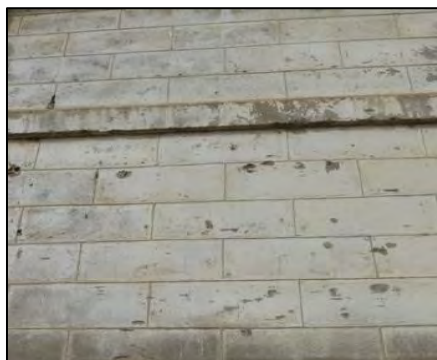
Photograph 18. Bldg. 4-Section of concrete-block wall.
