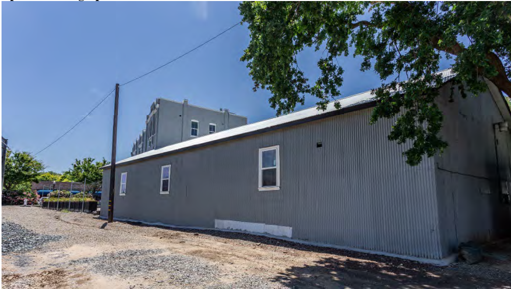
Photograph 1. View southwest of the north and east elevations.
