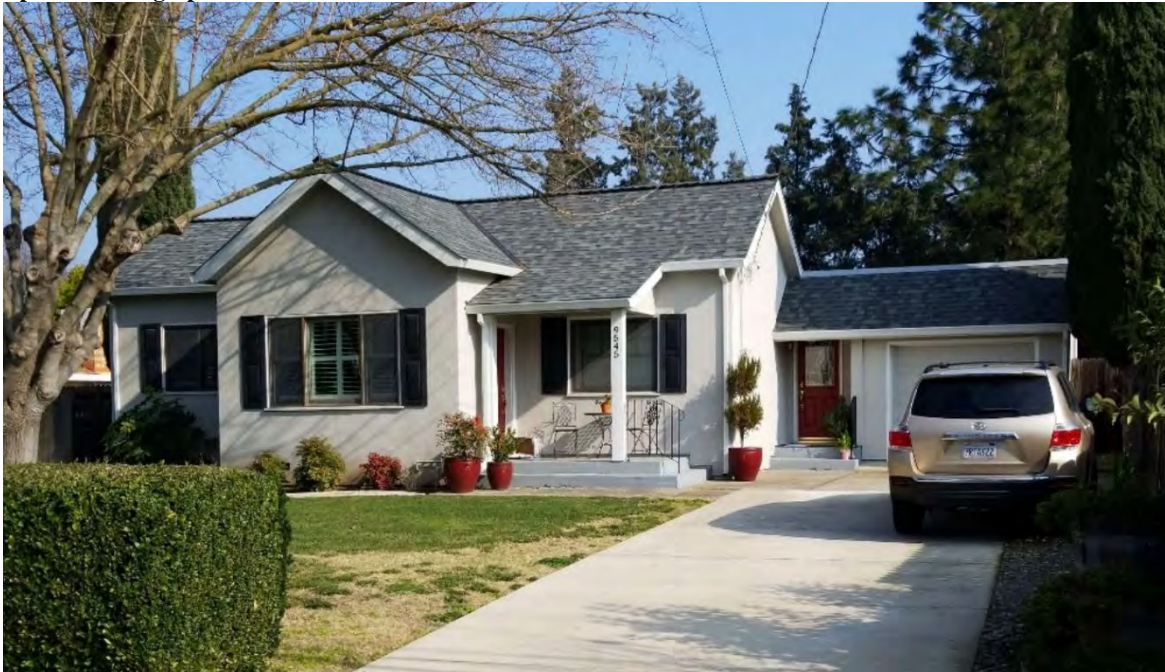
Photograph 1. View northeast of the west elevation.
