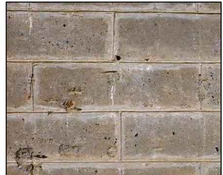
Photograph 19. Bldg. 4-Closeup of original concrete block wall.
