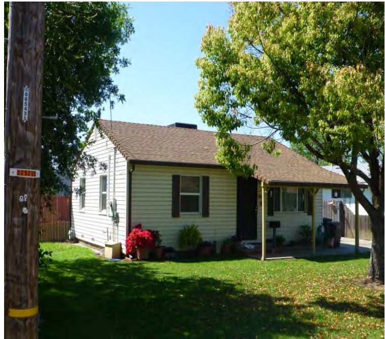
Photograph 2. View southwest of north and east elevations.
