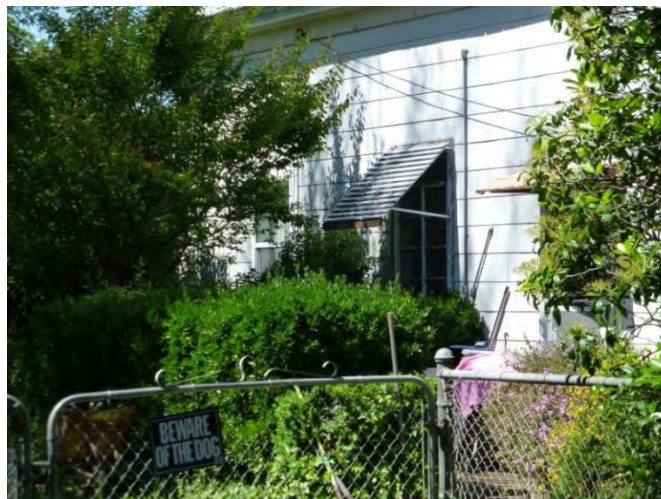
Photograph 2. View northwest of south elevation.
