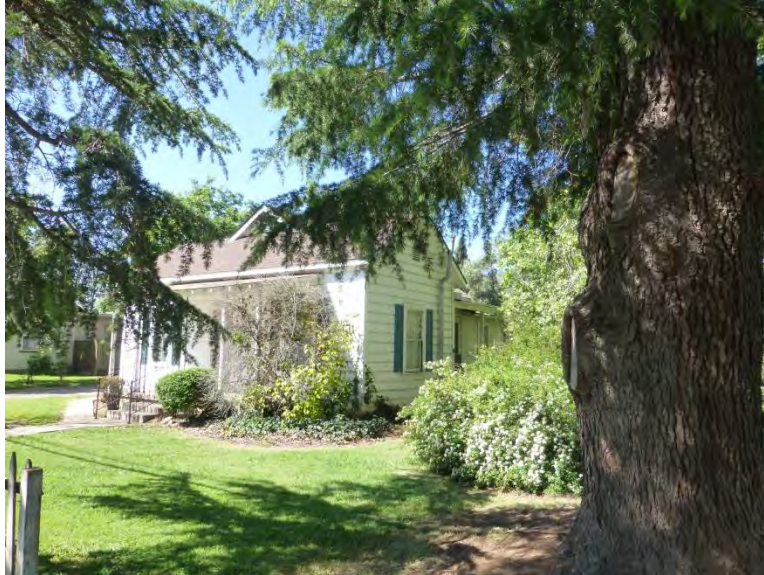
Photograph 2. View southwest of north and east elevations. Taken 4/10/14, # 0643.
