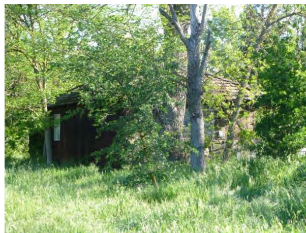
Photograph 6. West & south elevations of detached garage. Camera facing northeast.
