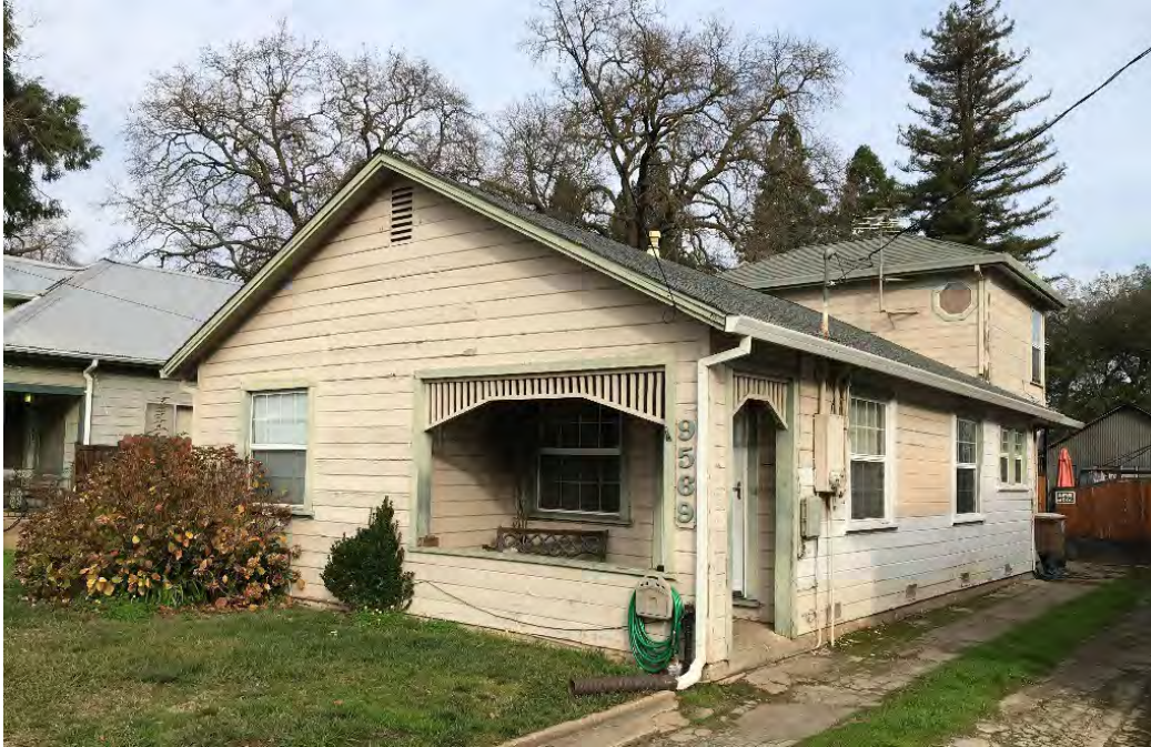
Photograph 1: View northeast of west and south elevations.
