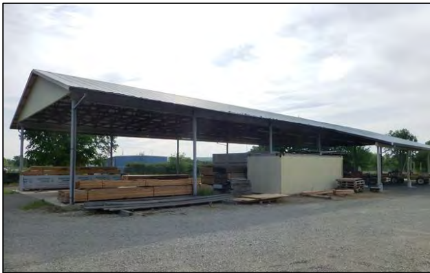
Photograph 9. West & north elevation of non-contributing pole barn.
