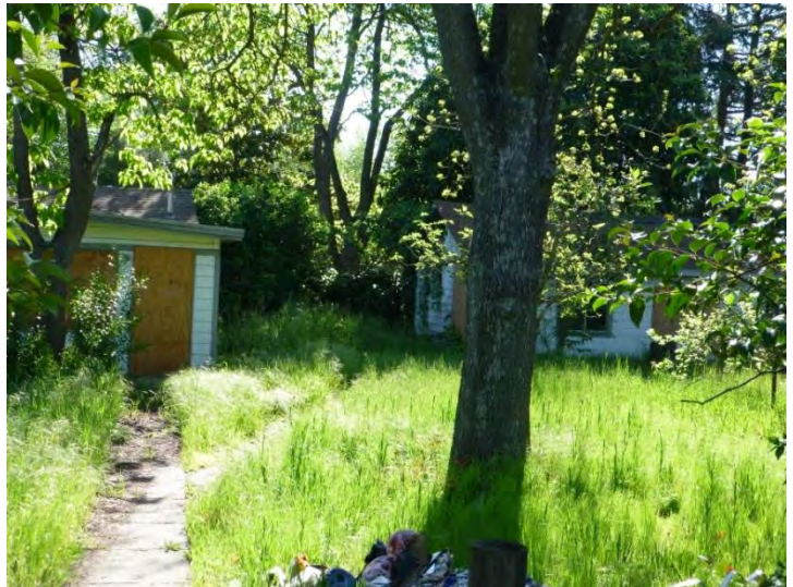
Photograph 2. View southeast of ancillary building. Taken 4/10/14..
