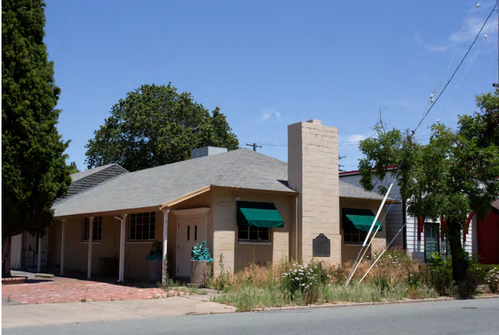
Photograph 1. View northeast of the west and south elevations.
