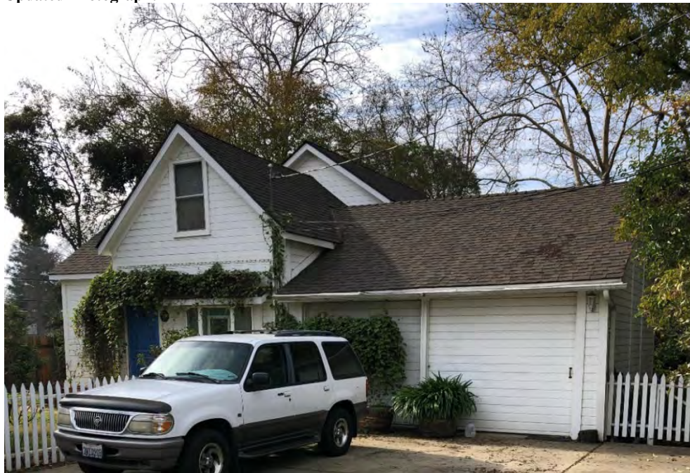
Photograph 1. View southwest of the east elevation.
