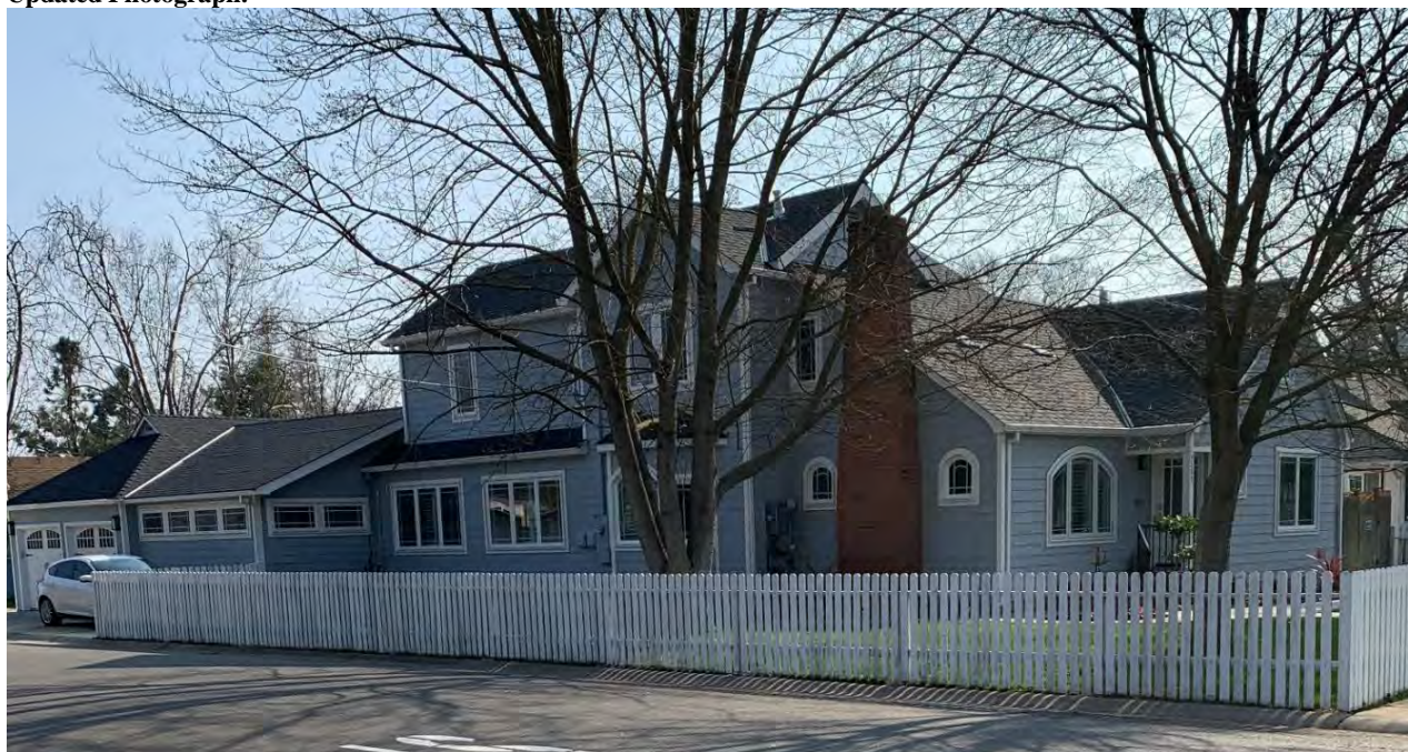
Photograph 1. View southwest of the north and west elevations.
