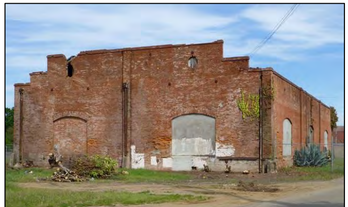
Photograph 3. South and east elevations. Camera facing northwest.
