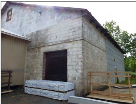
Photograph 17. Bldg. 4-north & west elevations of winery warehouse.
