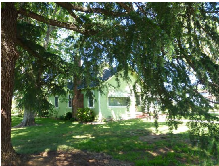
Photograph 3. View northwest of south and east elevations. Note the exterior brick chimney. Taken 4/10/14, #0642.
