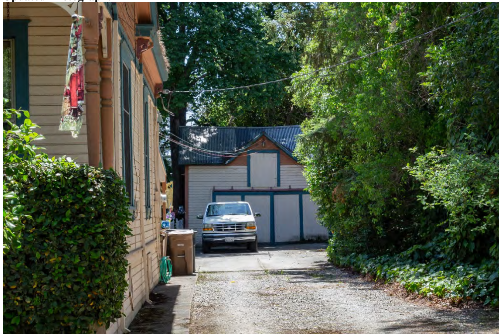
Photograph 1. View south of the north elevation.
