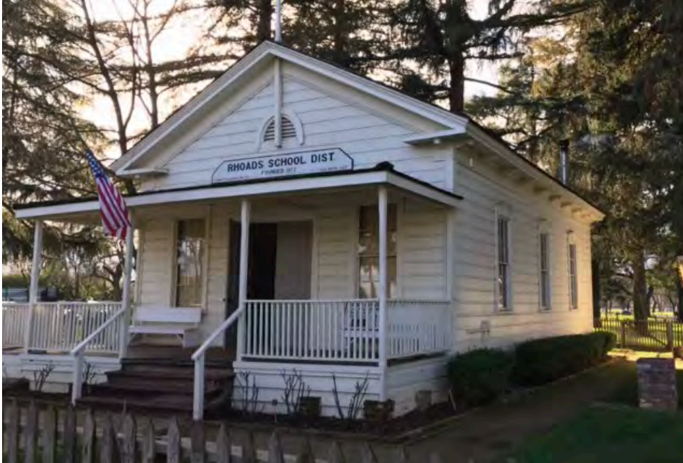
Photograph 1. View north of east and north elevations.
