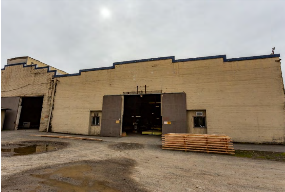
Photograph 3. View southwest of the north elevations of Building 6 and 5.
