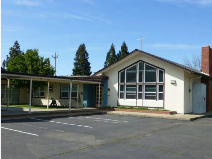
Photograph 4. View northwest of education building.
