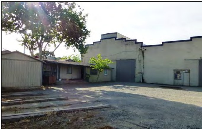
Photograph 1. Left to right: Non-contributing office building constructed in 1972 and enlarged in 1979; north elevation of Bldg. 6; and east half of north elevation of Bldg. 5.
