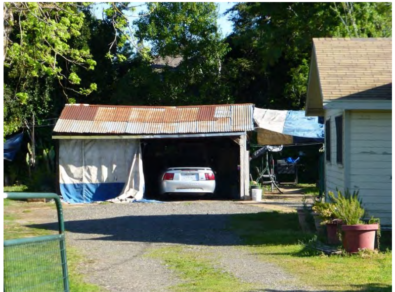
Photograph 2. View northwest of detached garage. Taken 4/10/14.
