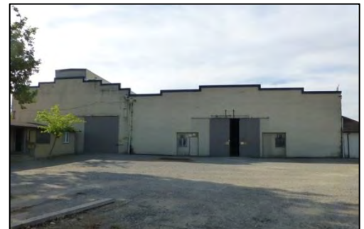
Figure 12. Bldg. 5-Storage Bldg. (right) and Bldg. 6-Bottling facility & Sherry Oven (left).
