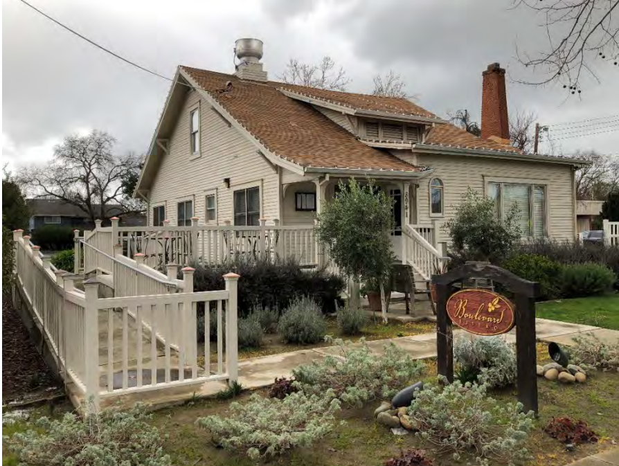
Photograph 1. View northeast of the west and south elevations.
