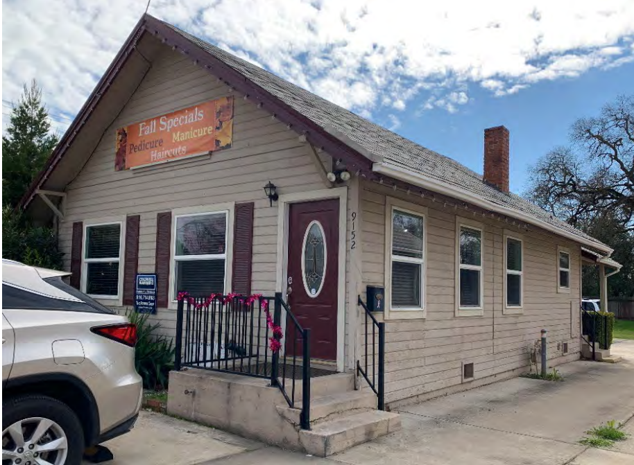
Photograph 1. View southeast of the north and west elevations.
