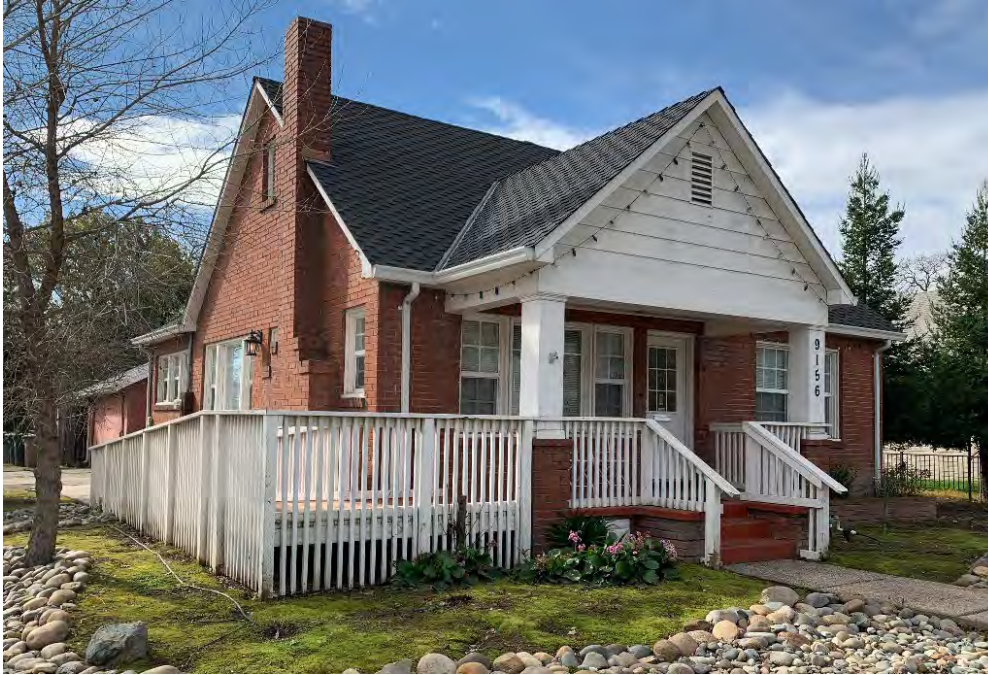
Photograph 1. View southwest of the north and east elevation.
