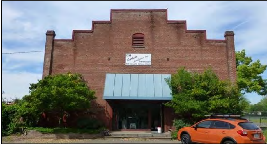
Photograph 2. Front façade (east elevation) of Elk Grove Winery Warehouse. Camera facing west.
