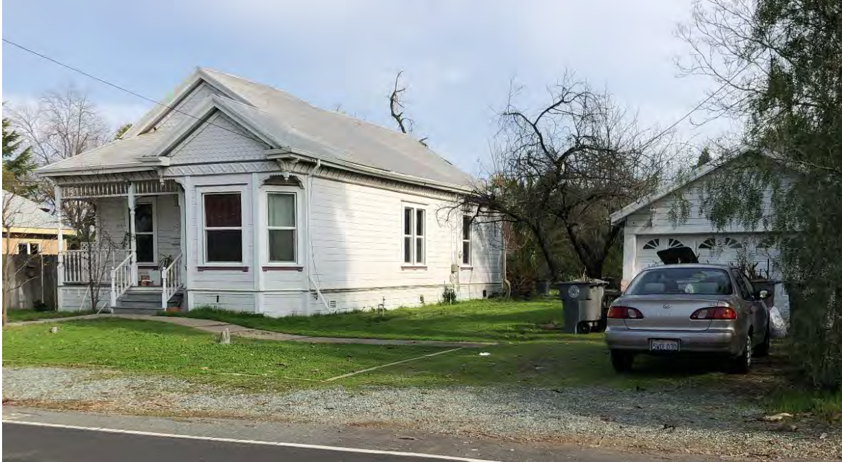
Photograph 1. View northeast of the west and south elevations.
