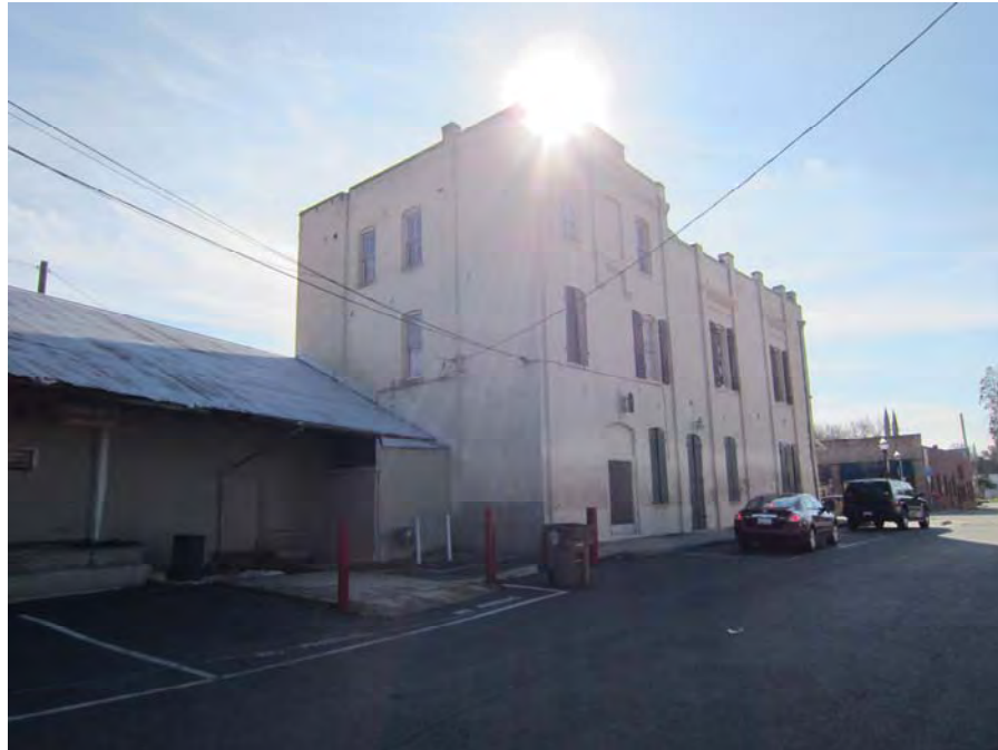
View of north and west facades of IOOF Building and adjoining warehouse building (Page & Turnbull, 02/13/2012).
