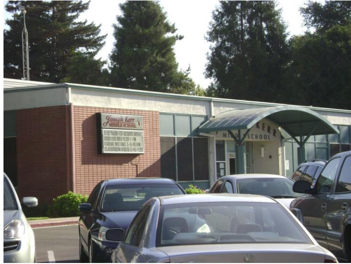
Joseph Kerr Middle School, 9965 Elk Grove Road. Photograph by Page & Turnbull, 2012.
