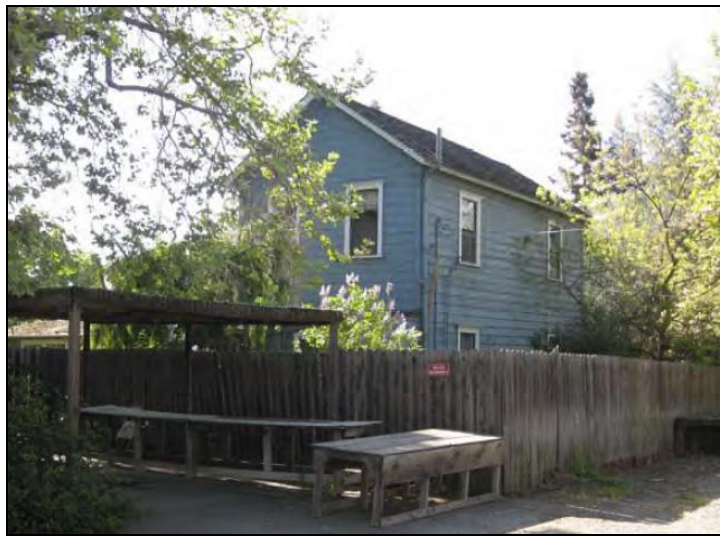
The Kirby Ranch house, built circa 1880 Photograph by Page & Turnbull, 2012.
