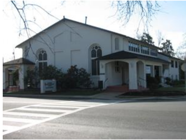
Community Methodist Church, 8986 Elk Grove Boulevard, looking south. Photograph by Page & Turnbull, 2012.
