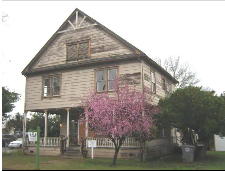
George Harvey Kerr house, built in 1859 The ground floor was raised circa 1885 to insert a new first story. Photograph by Page & Turnbull, February 2012.
