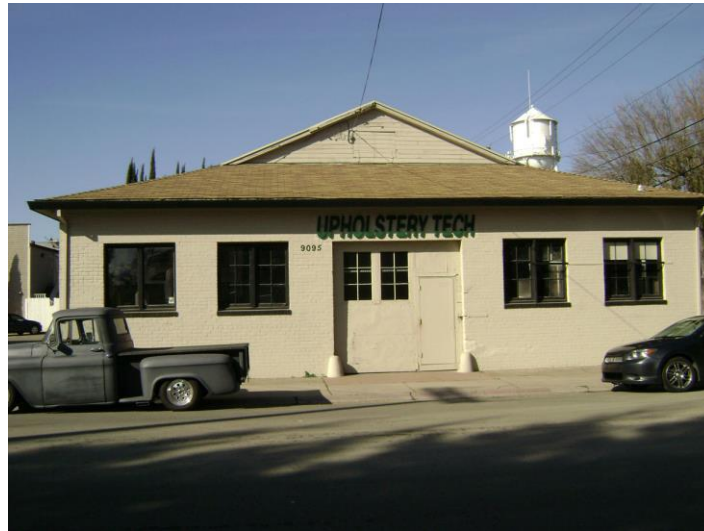
Batey Garage, 9095 Elk Grove Boulevard, looking north. Photograph by Page & Turnbull, 2012.
