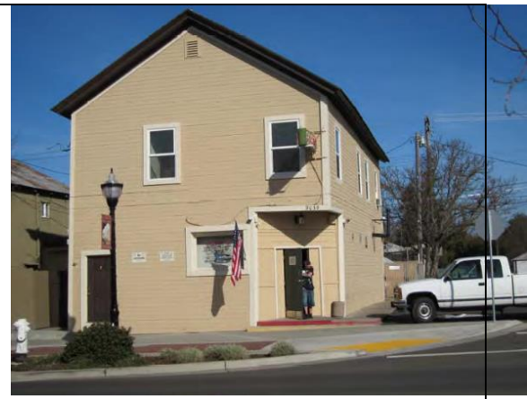
Bob’s Club, formerly the Elk Grove Hotel at 9039 Elk Grove Boulevard. Photograph from Page & Turnbull, 2012.
