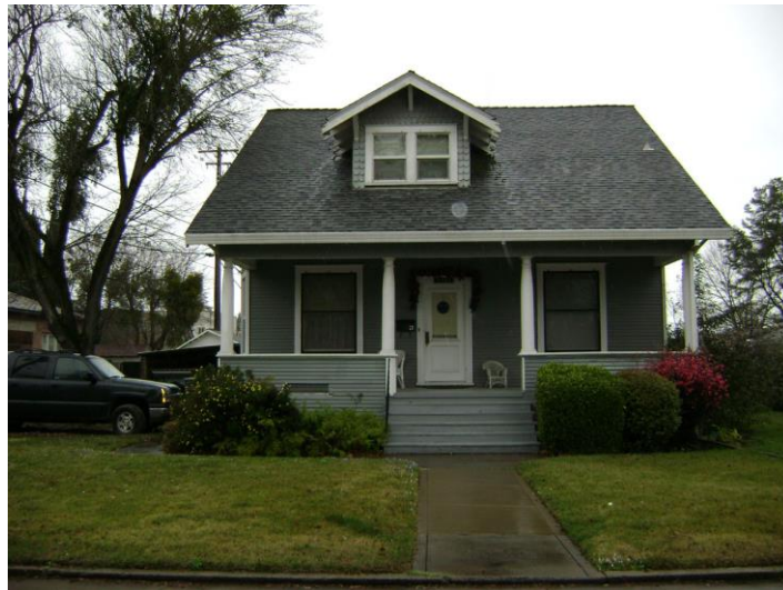
Ira Jones House, 9588 School Street, looking west. Photograph by Page & Turnbull, 2012.
