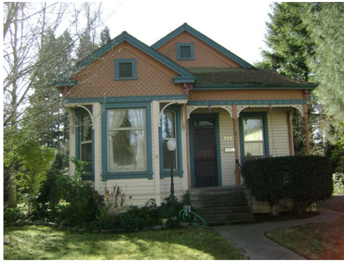
Brainard/Markofer Residence, 9112 Elk Grove Boulevard, looking south. Photograph by Page & Turnbull, 2012.
