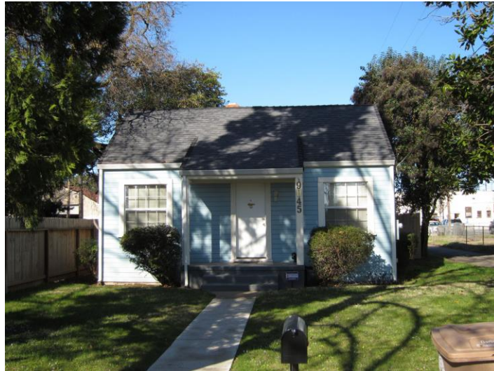
Brill Residence, 9045 Grove Street, looking north. Photograph by Page & Turnbull, 2012.
