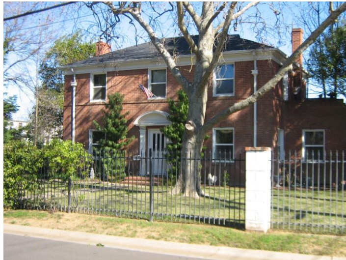
Judge Godfrey and Marion Mix House, 9565 School Street, looking east. Photograph by Page & Turnbull, 2012.
