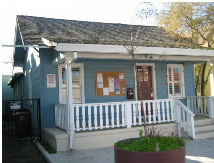
Hayes Residence, 9030 Elk Grove Boulevard, looking south. Photograph by Page & Turnbull, 2012.
