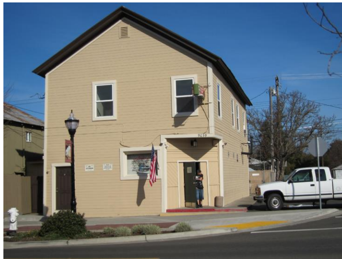
Bob’s Club, 9039 Elk Grove Boulevard, looking north. Photograph by Page & Turnbull, 2012.
