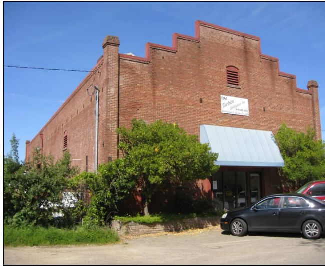
The former Elk Grove Winery warehouse, constructed in 1905 at 9678 Railroad Street. Photograph from Page & Turnbull, 2012.
