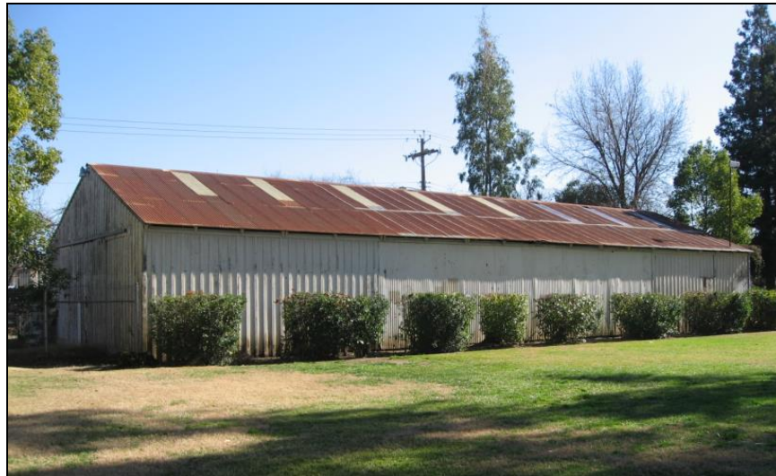
The former Williamson packing shed built in 1944 and located behind the Senior Center of Elk Grove. This appears to be the last remaining fruit packing shed located in Elk Grove. Photograph from Page & Turnbull.
