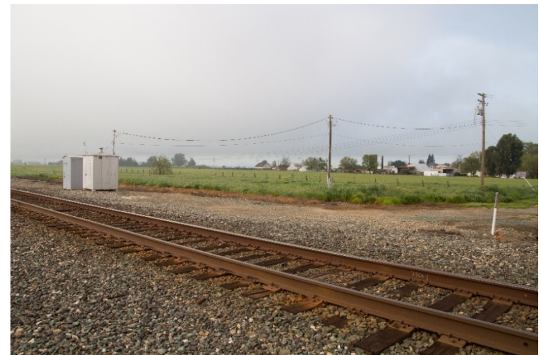
Looking southwest from railroad at Bilby
