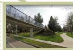
Grade-Separated Shared-Use Crossing
