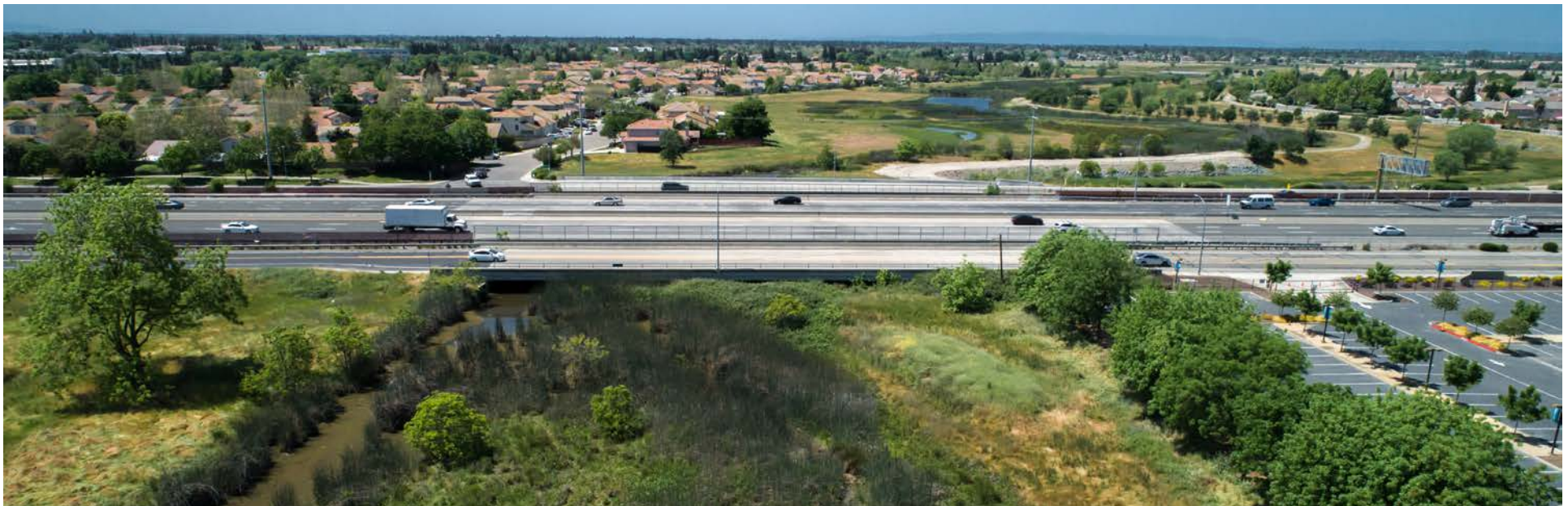
State Route 99 bridge over Laguna Creek.
