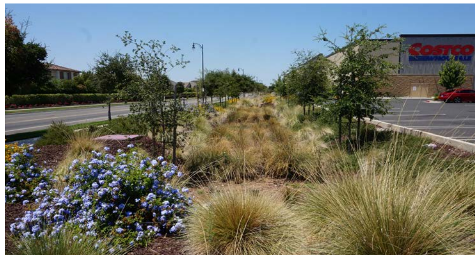
Bioswales and other green infrastructure can help reduce localized flooding impacts, improve water quality, and mitigate the UHI effect.
