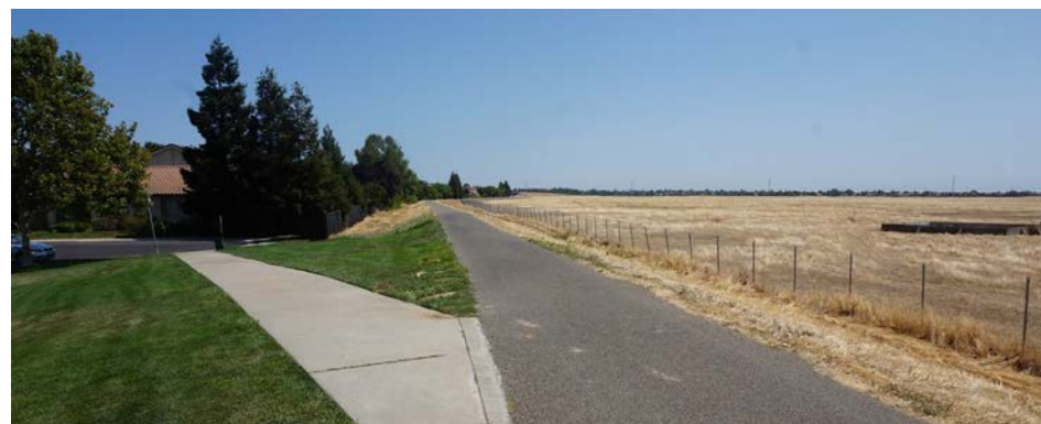
Laguna West Levee in Elk Grove at Don Nottoli Park"
