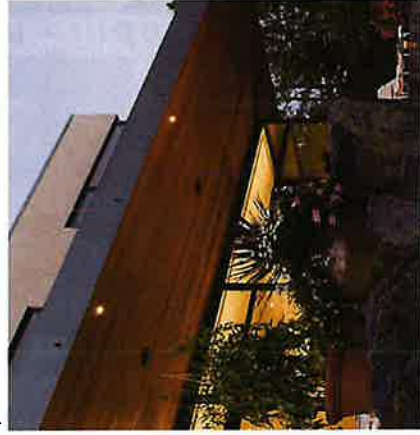
Small recessed downlights along guest path at Animal Care viewing windows. Downlights to have deep regressed apatured lighting to reduce lighting glare on glass.
