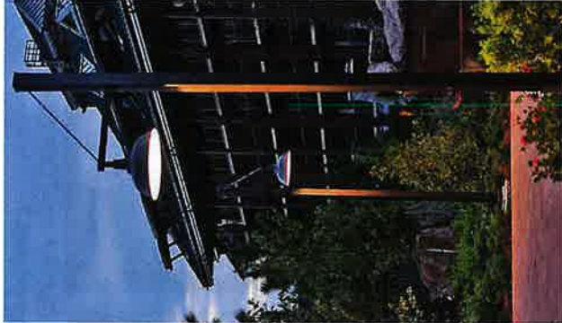
Pole mounted RLM shades for general illumination in open areas.
