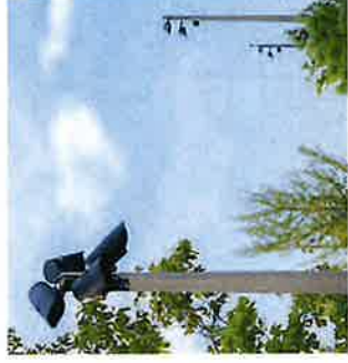
Habitat illumination via shade structure mounted gobo projectors with visors. Where surrounding structures are not tall enough and there are no appropriate trees for moonlighting, discrete poles with will be utilized for mounting.
