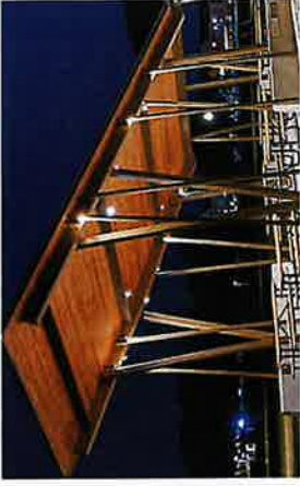
Surface mounted adjustable accents to illuminate pathways adjacent to shade structures.
