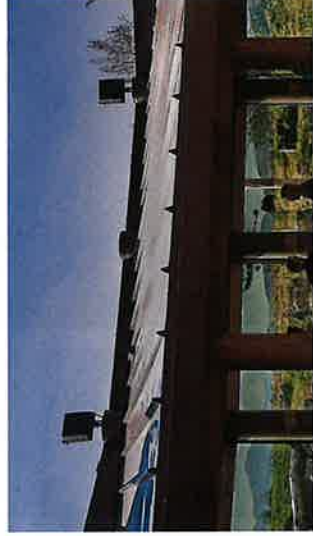
Habitat illumination via shade structure mounted gobo projectors with visors. Where surrounding structures are not tall enough and there are no appropriate trees for moonlighting, discrete poles with will be utilized for mounting.
