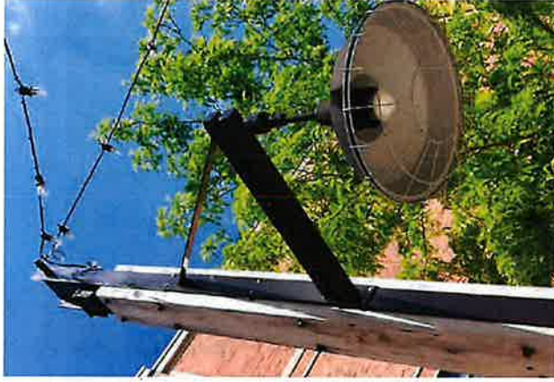
Pole mounted RLM shades for general illumination in open areas.
