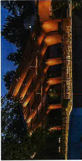
Surface mounted downlighting at viewing shade structures for general illumination.
