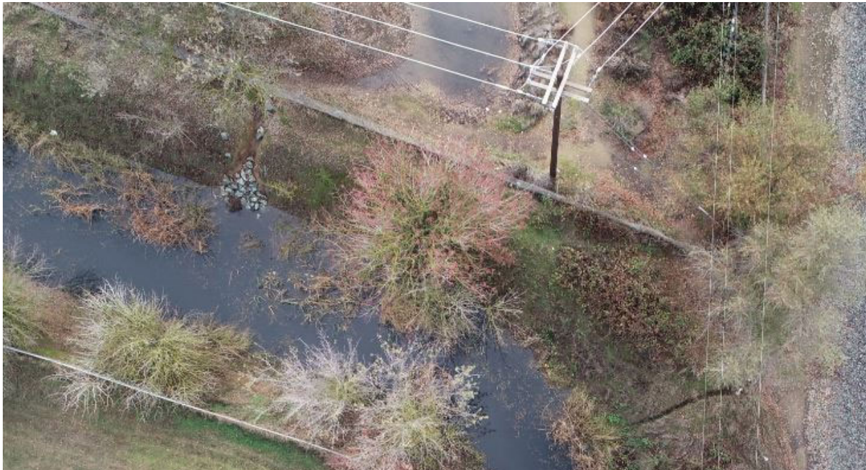
Figure 4 – Existing Berm located on Elk Grove Creek
