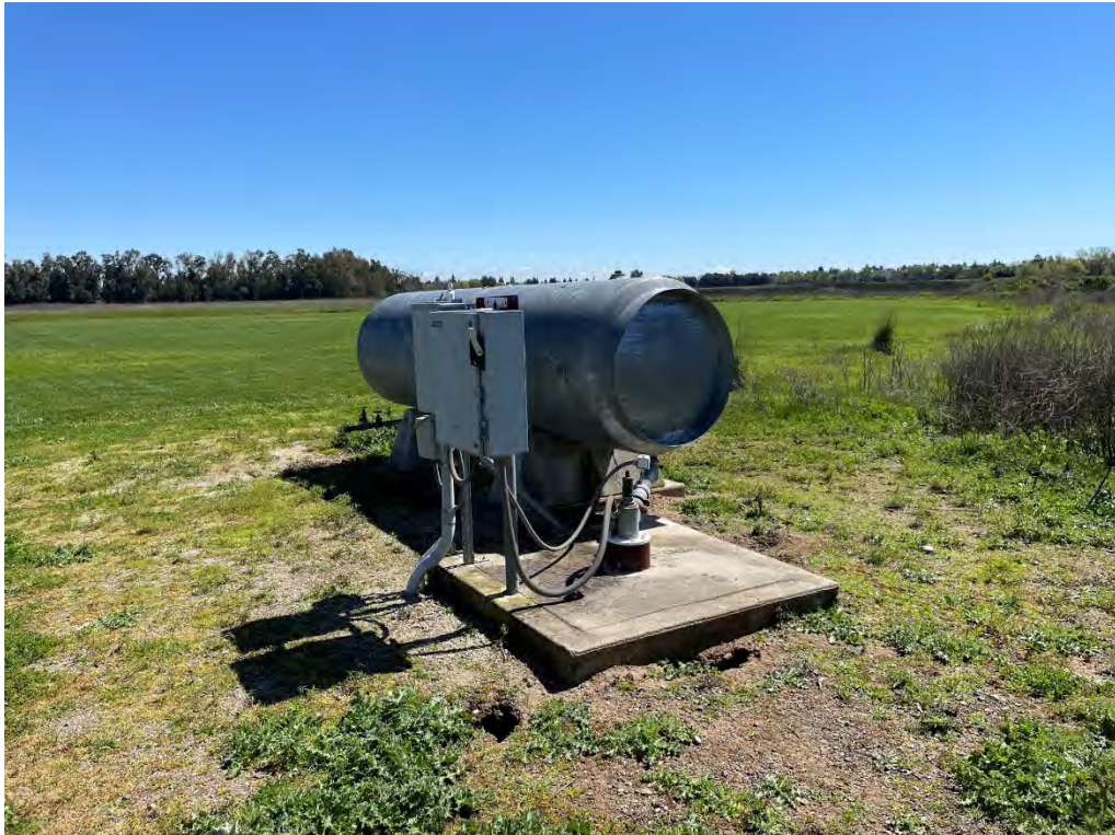
Photo No. 14 Irrigation water supply well and water aboveground storage tank in the offsite area within the eastern portion of the Project Study Area
