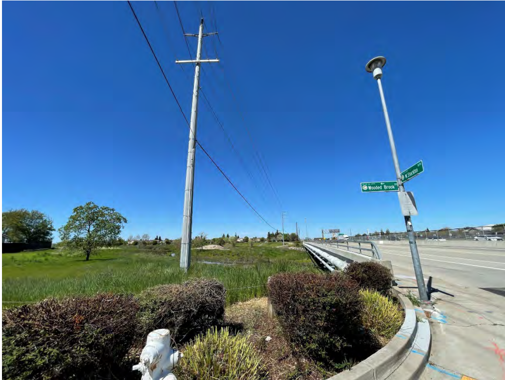
Photo No. 15 Electrical transmission line along West Stockton Boulevard from the western portion of the Project Study Area
