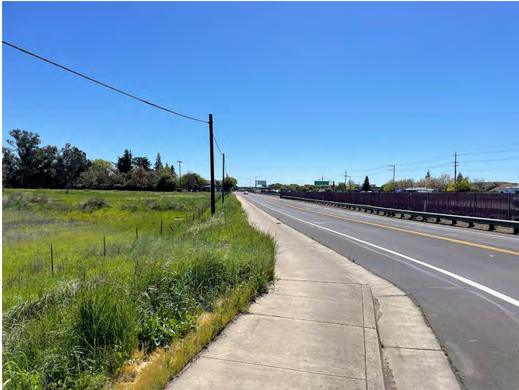
Photo No. 20 View to the south of the continuation of East Stockton Boulevard from the southern boundary of the Project Study Area
