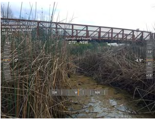
Laguna Creek – East end facing east
